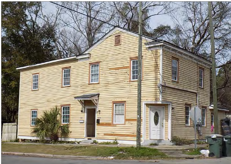
Figure 21. 802 W. 41 st Street (c1903), GNAHRGIS #8436 – Carpenter Italianate.
