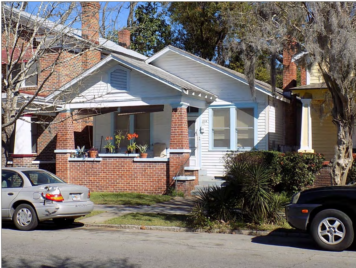
Figure 41. 614 W. 40 th Street (c1920), GNAHRGIS #8577 – The front gable bungalow is the most common subtype found in the survey area as well as the most common building type overall.
