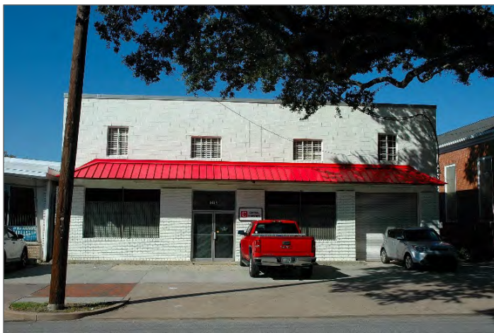
Figure 72. 1415 MLK, Jr. Blvd. (c1956), GNAHRGIS #268040. Mid 20 th Century iteration of the retail and office type commercial building.
