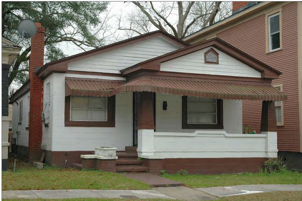
Figure 43. 711 W. 42 nd Street (c1940), GNAHRGIS #262453 – One of several concrete block, mid-20 th century examples within the survey area.
