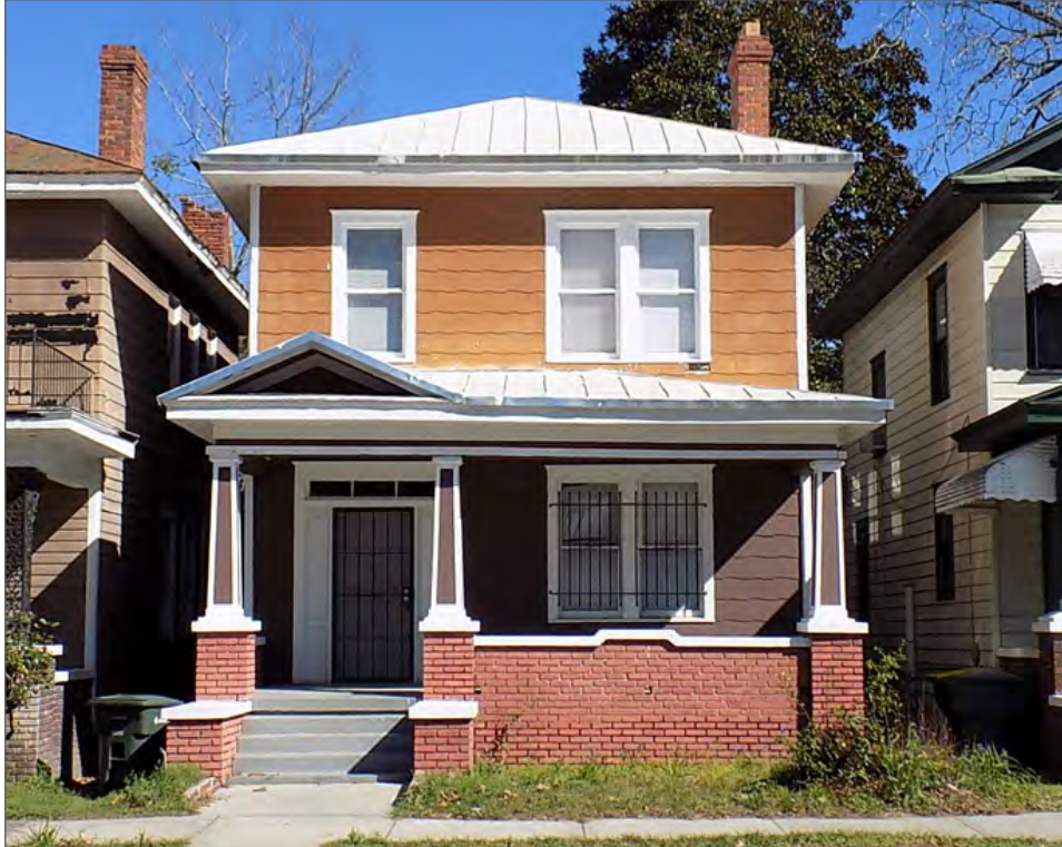
Figure 53. 622 W. 40 th Street (c1916), GNAHRGIS #8573 – Most examples of the American Foursquare type that were identified during the survey are more rectangular in shape – like this example.
