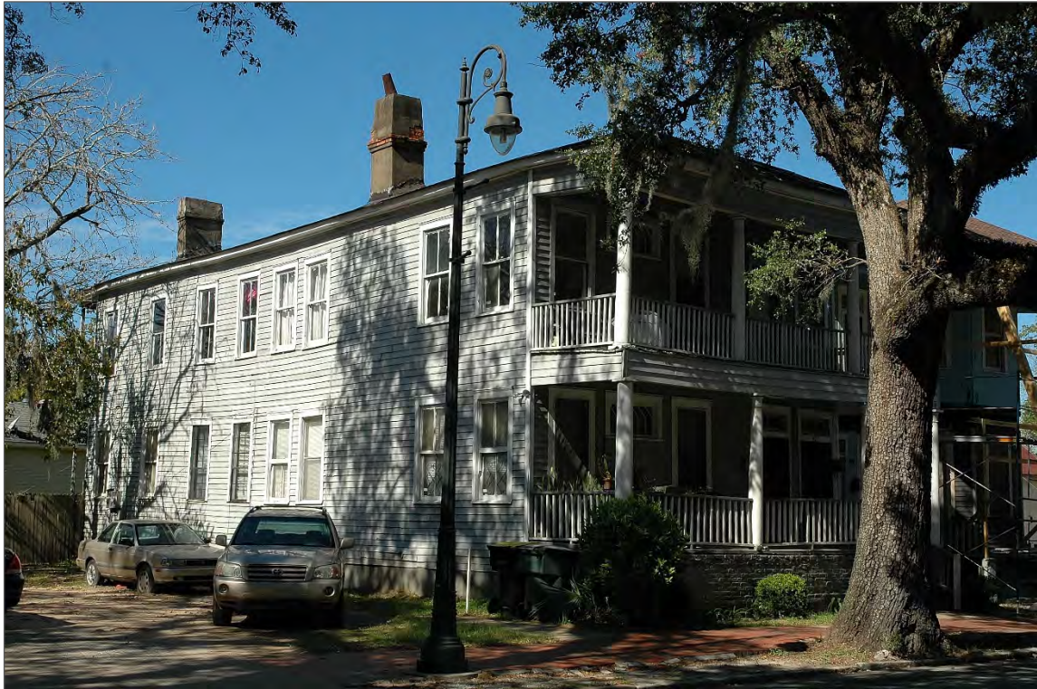
Figure 63. 1817-1817 ½ MLK, Jr. Blvd. (c1907), GNAHRGIS #8133 – An early example of a duplex house in the neighborhood – note separate entry doors and recessed portico supported by round Tuscan columns.
