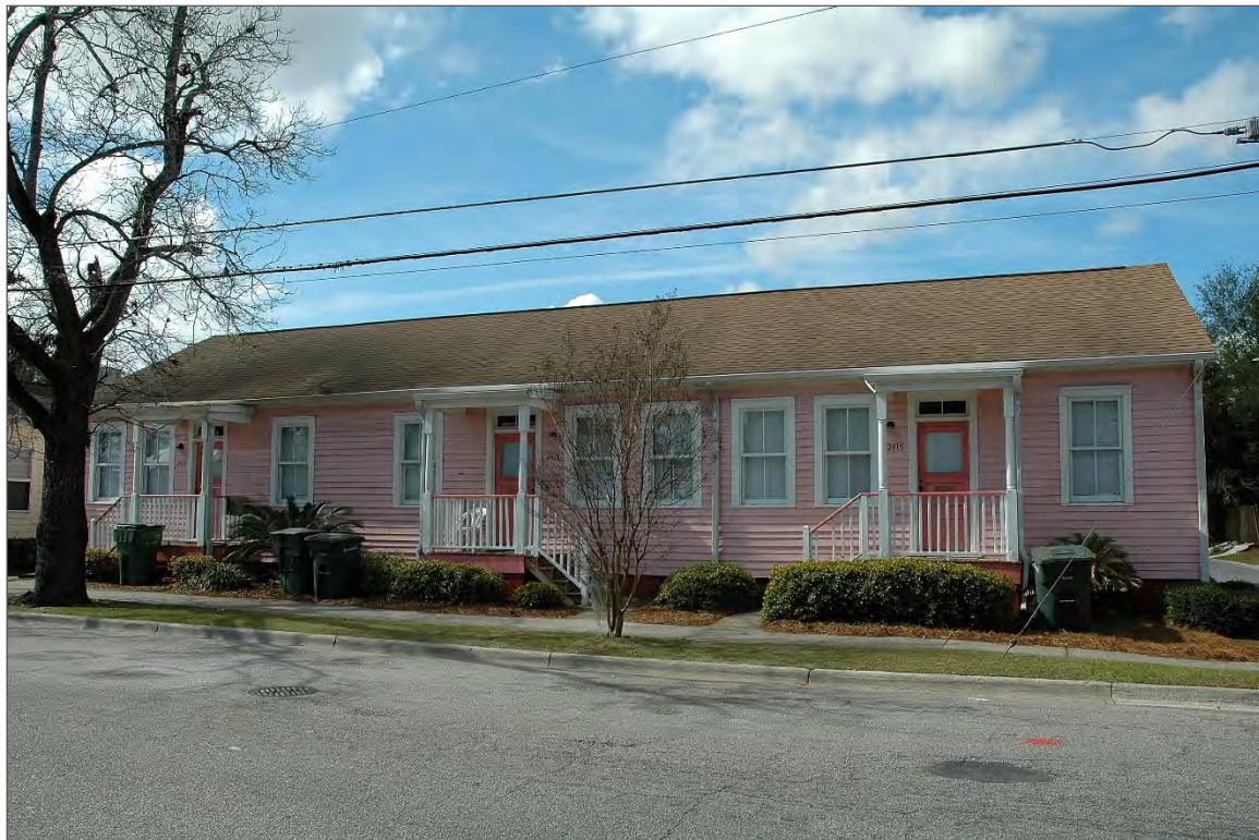
Figure 35. 2415-2419 Burroughs Street (c1912), GNAHRGIS #8593 – A three-unit, one-story rowhouse with a four-square plan – one of eleven examples within the district that contain between three and five separate living units.
