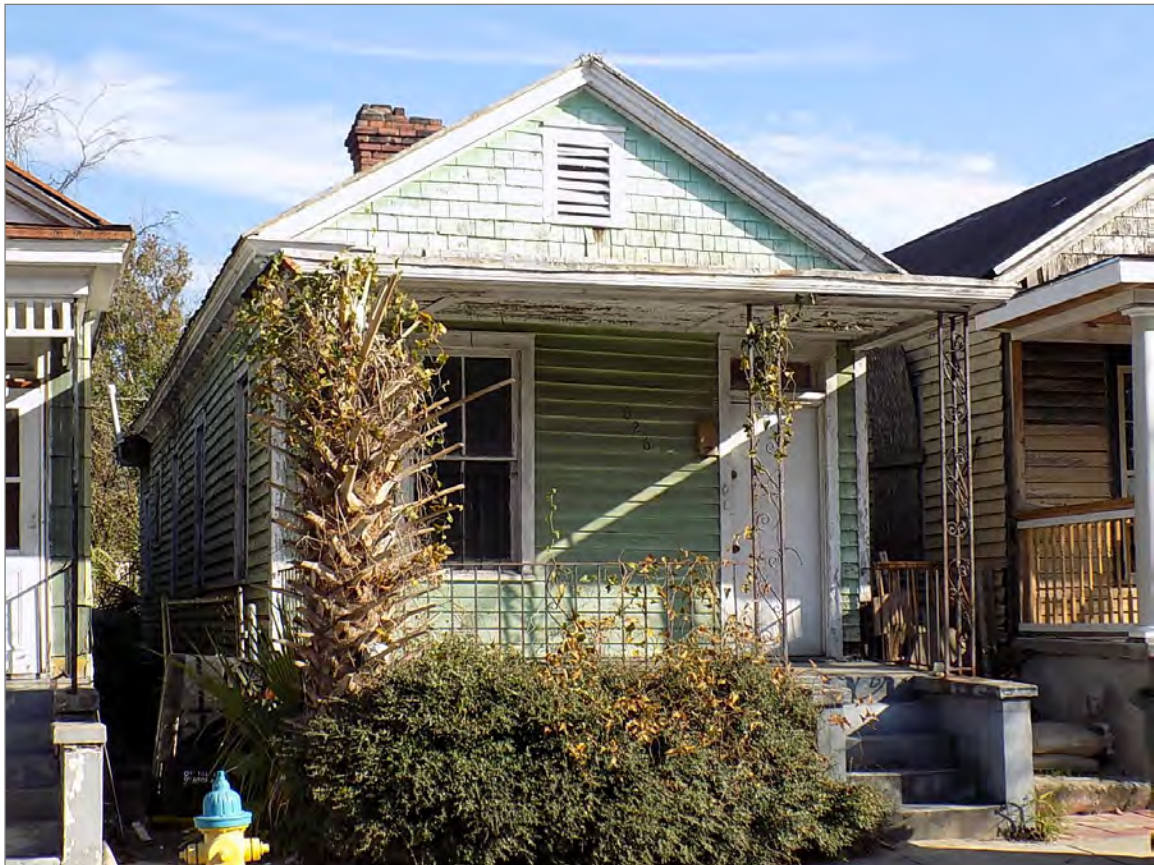
Figure 38. 626 W. 42 nd Street (c1901), GNAHRGIS #8617 – One of a row of fifteen identical shotgun houses.
