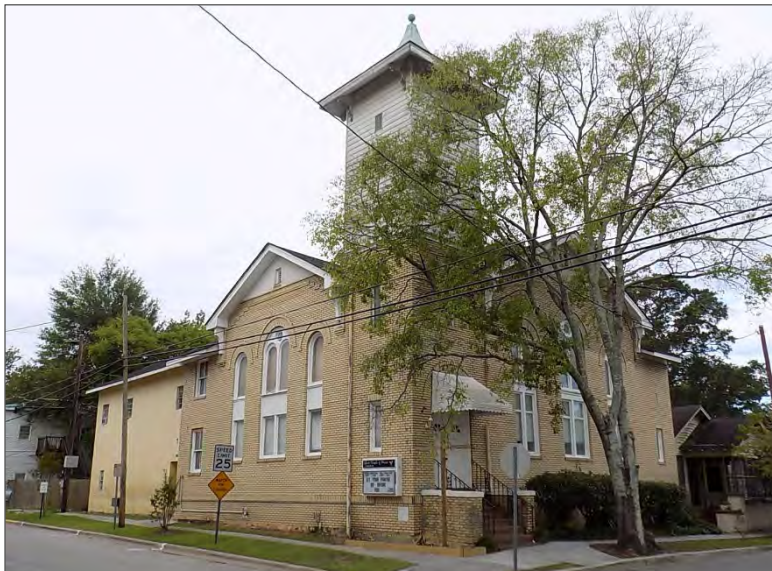
Figure 68. Palen Methodist Episcopal Church (c1920), GNAHRGIS #268043. A substantial corner tower example displaying elements of the Romanesque and Italianate styles.
