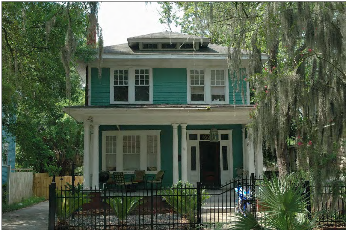
Figure 52. 609 W. 37 th Street (c1916), GNAHRGIS #8503 – Prairie style American Foursquare, typical of the more substantial examples found in the survey area.
