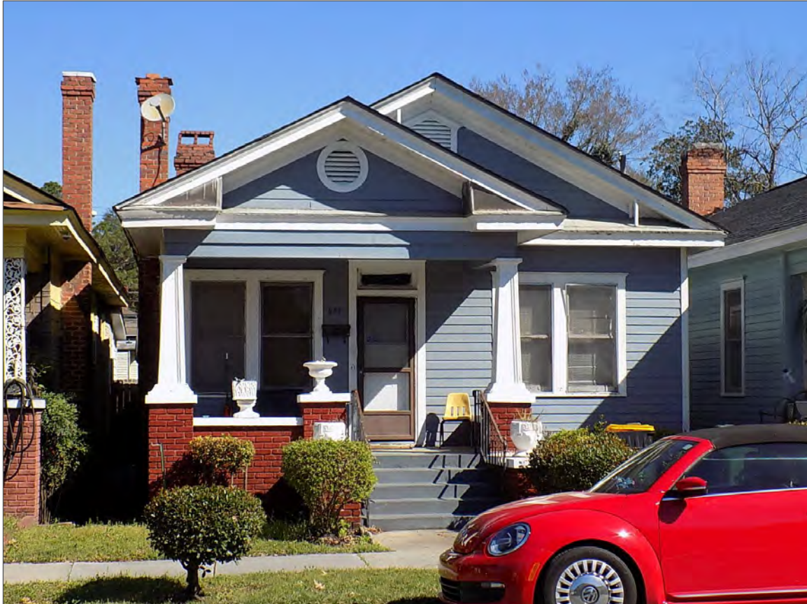
Figure 26. 632 W. 40 th Street (c1917), GNAHRGIS #8568. This example features Craftsman style columns in place of classical columns yet still evokes a strong sense of the Colonial Revival style in its pedimented front gable, gable portico with distinct entablature, round wood vent, gable return, supported by columns resting on brick piers, and one-light transom over door.
