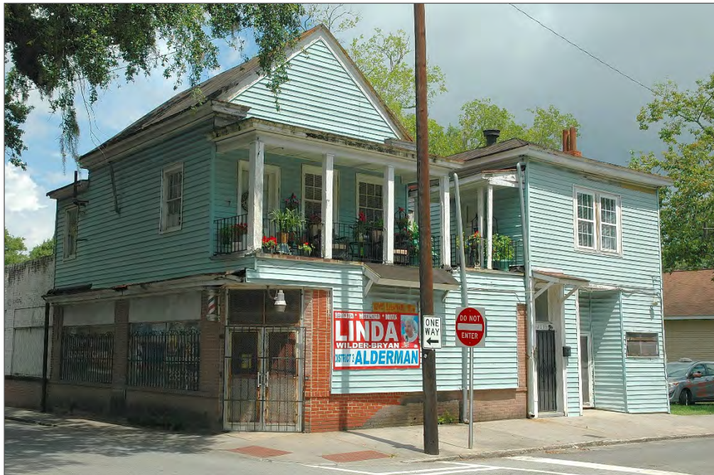
Figure 61. 2015 Florance Street (c1921), GNAHRGIS #8363 – An unusual example as the older shotgun house was raised a full story in order to build the commercial ground level c1921.
