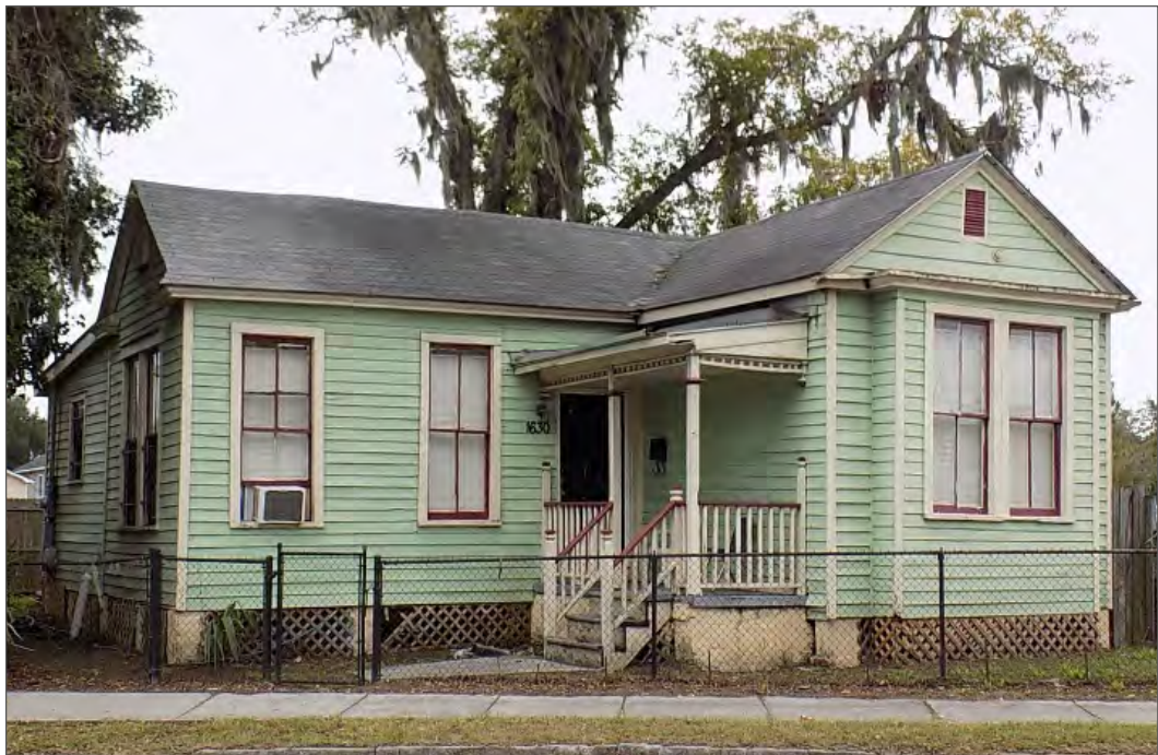
Figure 77. 1630 Ogeechee Road (c1910), GNAHRGIS #8058. One of three gable wing cottages. T or L-shaped, this three-room house features a gable front at one end and a recessed wing that is parallel to the façade.
