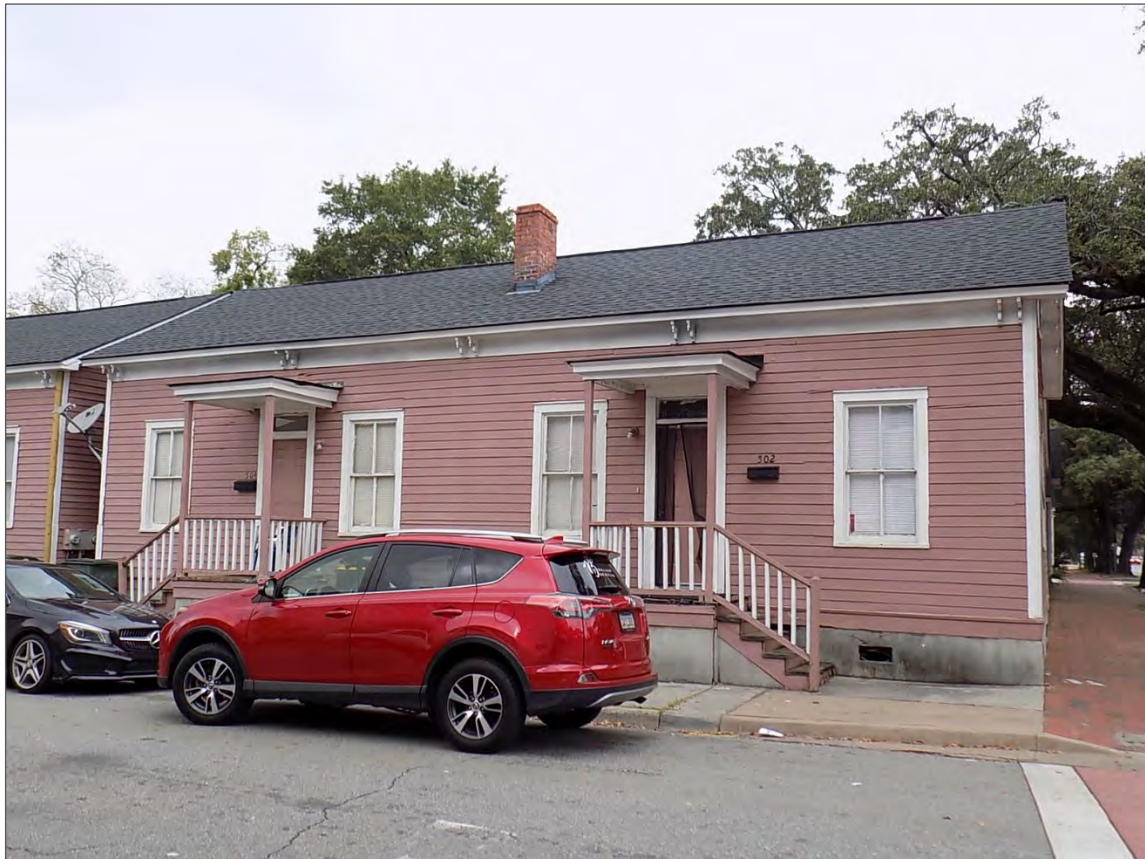
Figure 62. 502-504 W. 34 th Street (c1910), GNAHRGIS #8117 – An early example of a duplex cottage in the neighborhood – one of a series of five identical buildings along the block face.
