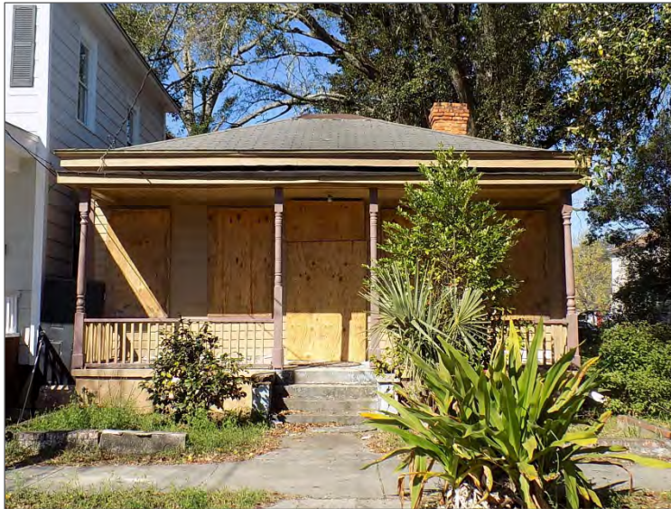
Figure 19. 2309 Florance Street (c1905), GNAHRGIS #8416 – This simple Georgian cottage type house displays very little ornament and – like almost 65% of buildings surveyed during the Cuyler-Brownville Neighborhood Historic Resources, is not a good representative example of an academic style. Therefore, this building is recorded in the survey inventory as having “no academic style” despite the presence of turned porch posts – which represents “elements” of the Folk Victorian style.
