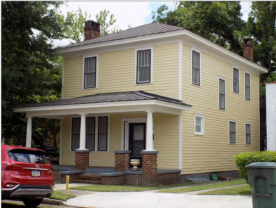
Figure 54. 909 W. 36 th Street (c1920), GNAHRGIS #8207 – a simple example of the type.
