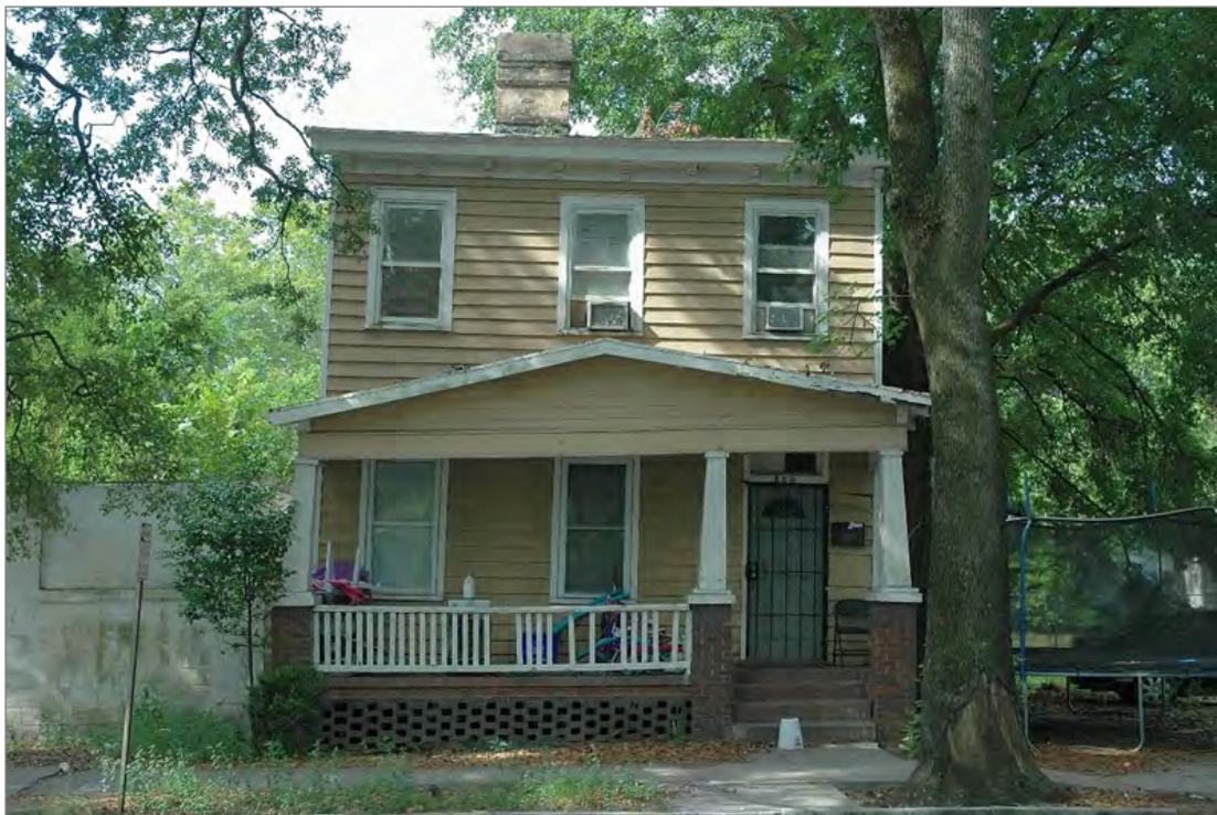
Figure 51. 809 W. 37 th Street (c1900), GNAHRGIS #8365 – A side gable example.
