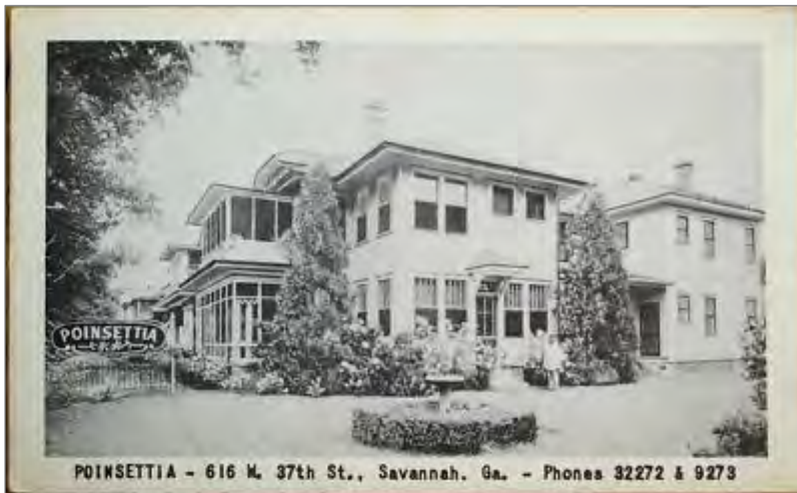
Figure 17. Circa 1940s postcard of the Poinsettia (tourist home) at 616 West 37 th Street. This building was demolished for a more modern tourist court (c1945) of the same name (GNAHRGIS #266687).
