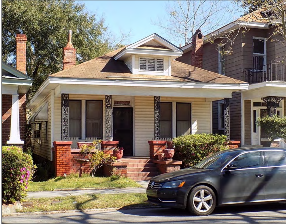
Figure 42. 626 W. 40 th Street (c1920), GNAHRGIS #8571 – An example of the hip bungalow subtype. This bungalow also exhibits the “Neoclassical Cottage” form, featuring a hip roof with boxed eaves, full width recessed porch (with columns originally), and pedimented façade roof dormer.
