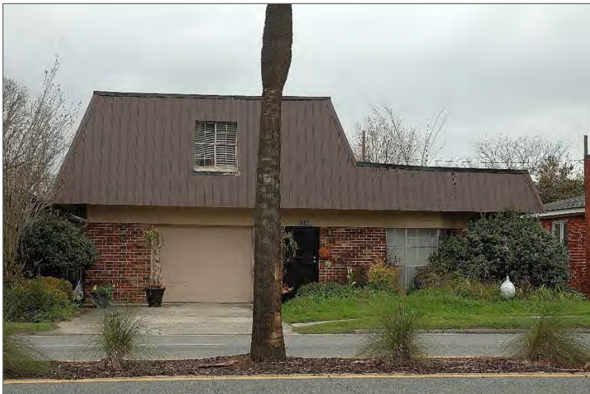
Figure 65. 1218 W. Victory Drive (1979), GNAHRGIS #271927 – This house is not representative of a building type recognized by the Historic Preservation Division.
