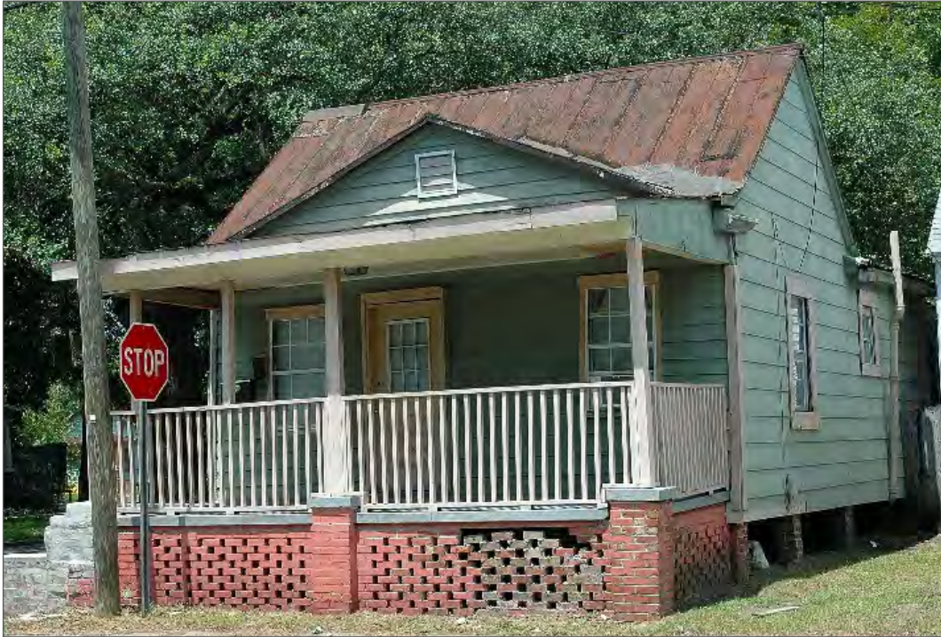
Figure 76. 2019 Harden Street (c1904), GNAHRGIS #8361. One of thirteen hall-parlor cottages identified within the survey area. Hall parlor houses feature two unequal rooms and are one room deep – entry is into the larger of the two rooms (parlor).
