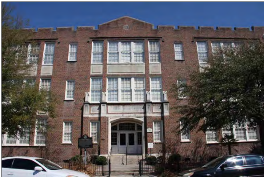
Figure 74. Florance Street School (c1928) – 700 W. 35 th Street, GNAHRGIS #8143. This example has an overall rectangular shape with shallow side wings that extend beyond the sides of the façade and rear elevation – almost giving it an H-shape. The building is a good example of Academic Gothic Revival.
