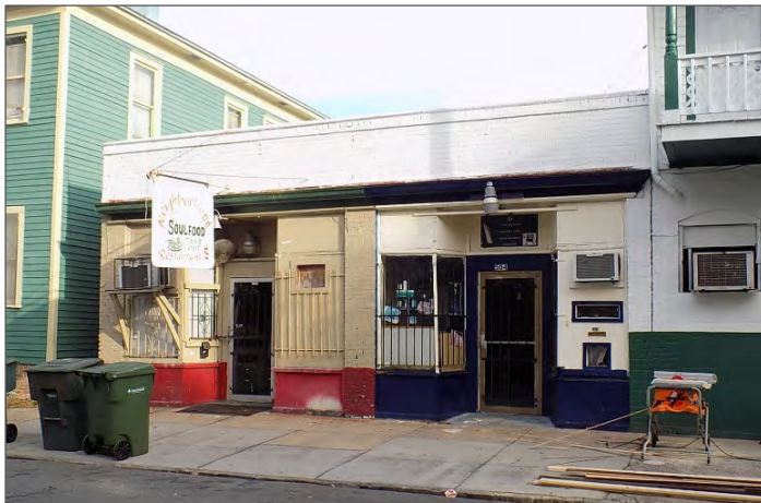
Figure 71. 504 W. 42 nd Street (c1922), GNAHRGIS #262488. Good example of a multiple retail type commercial building. This example is a more traditional iteration whereas most of the commercial type buildings in the survey are late period examples.
