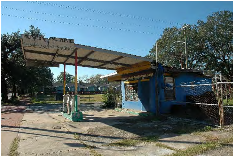
Figure 80. 1603 MLK, Jr, Blvd. (c1958), GNAHRGIS #268038. Mid-20 th Century, concrete block service station.
