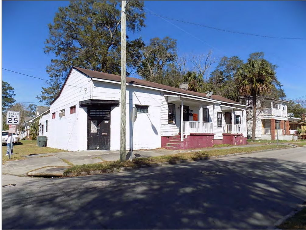
Figure 60. 2315-2319 Florance Street (c1908), GNAHRGIS #8426 – This cottage row is one of only two one-story examples identified within the survey area.
