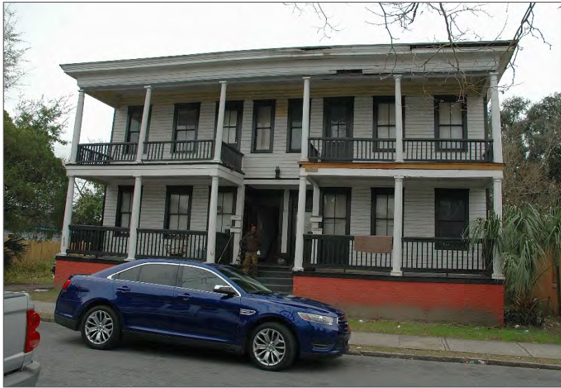
Figure 33. 617 W. 42 nd Street, GNAHRGIS #262501, typical balloon frame example built c1915.
