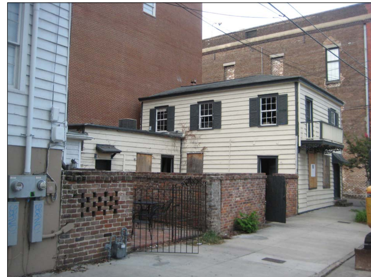
SIDE VIEW OF PROPERTY FROM LINCOLN STREET
