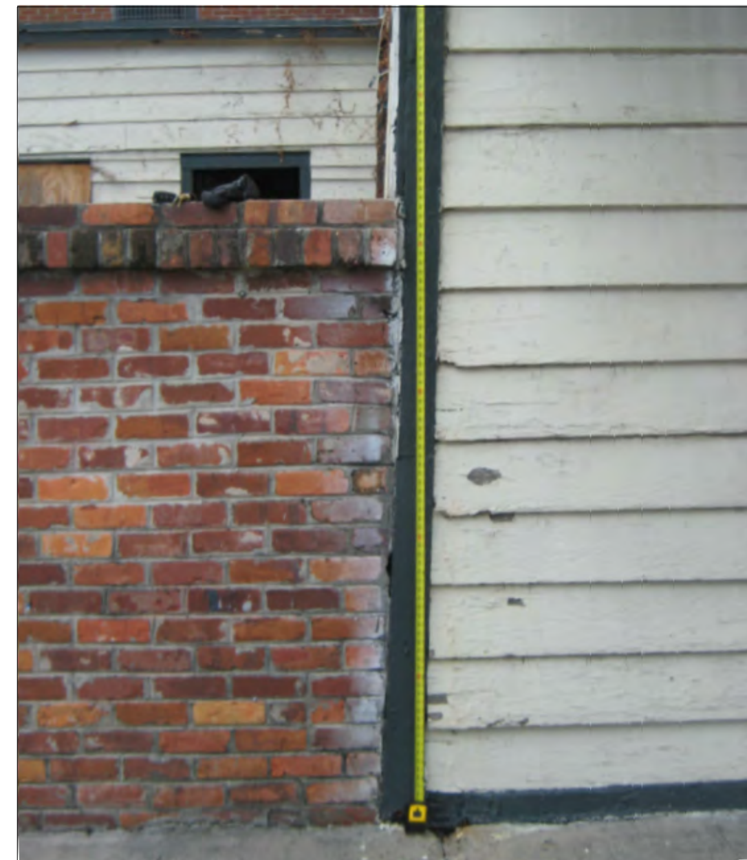
PLUMB LINE DROPPED FROM SECOND FLOOR - 6" OVERALL DIMENSION OUT OF LINE
