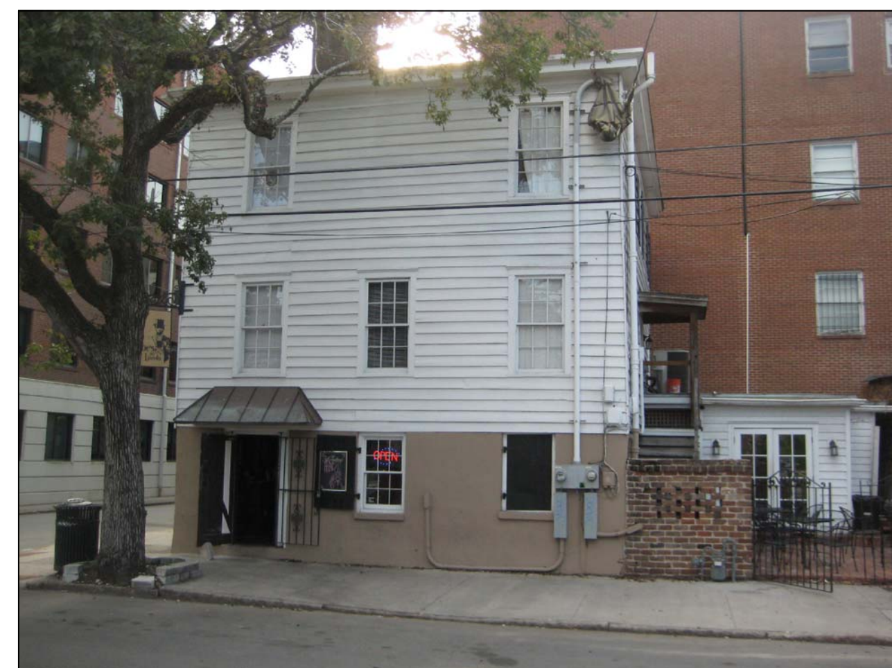
ADJACENT PROPERTY TO SOUTH ON LINCOLN STREET
