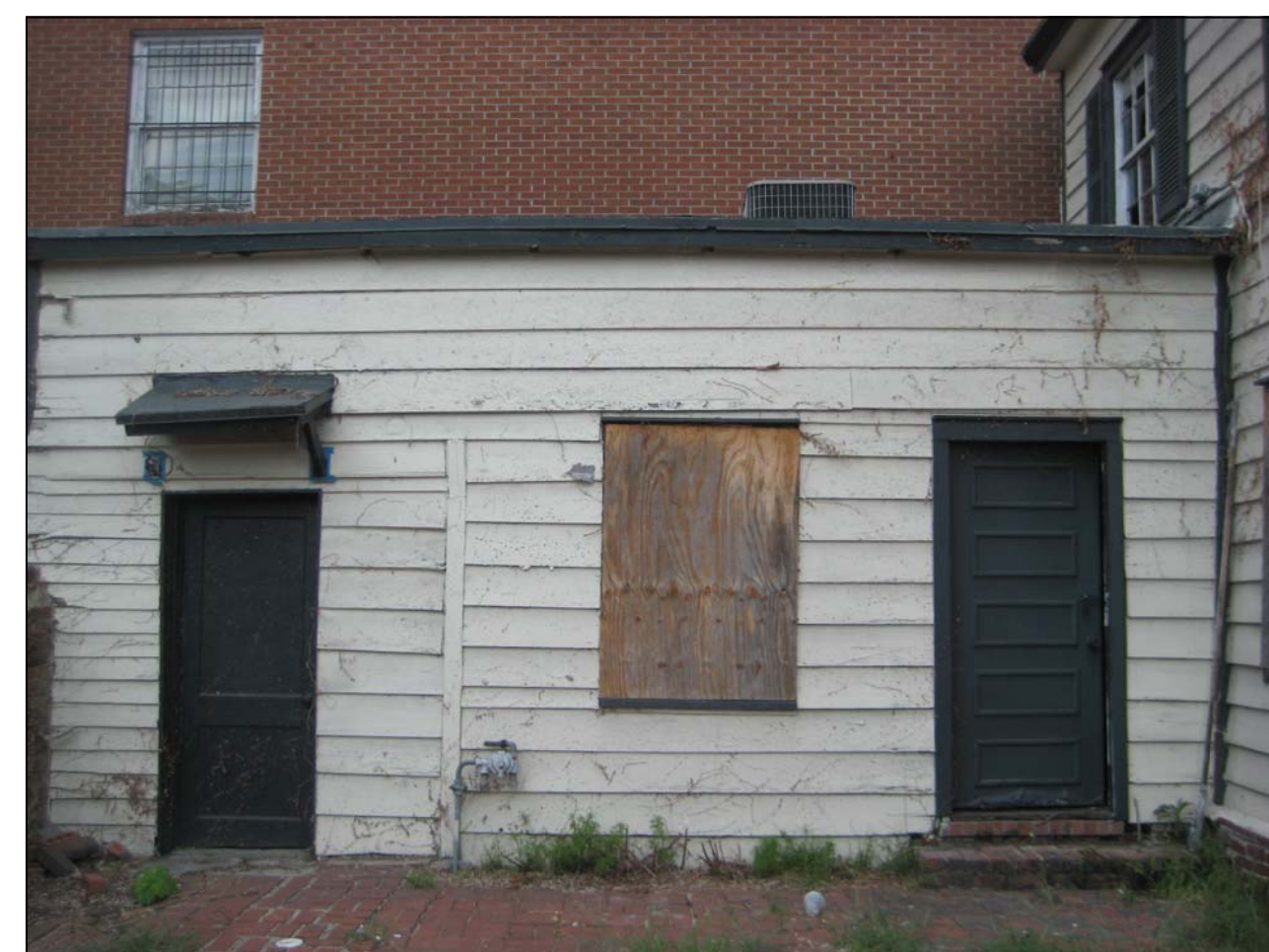
VIEW OF EXISTING SHED ADDITION FROM COURTYARD
