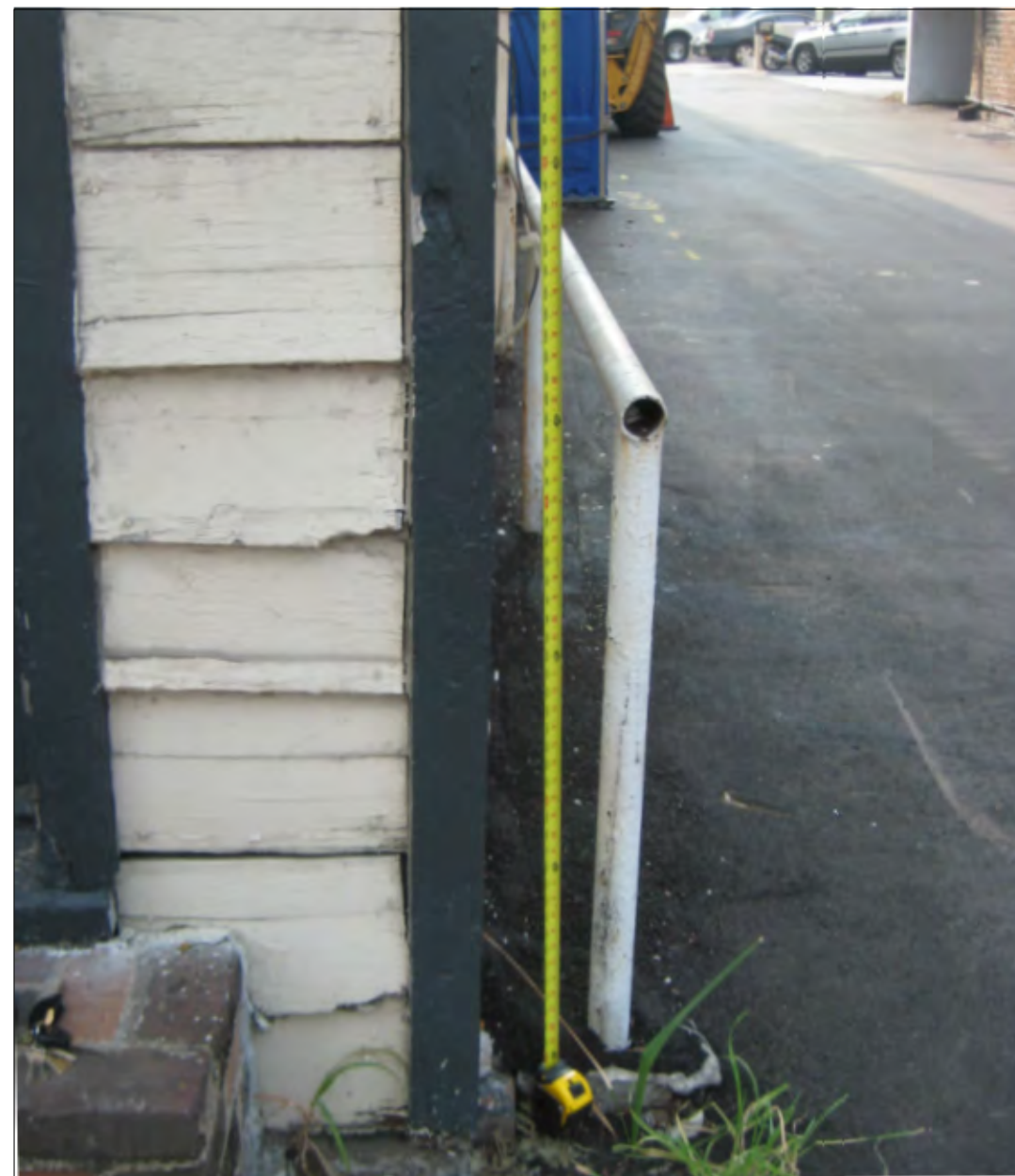
PLUMB LINE DROPPED FROM SECOND FLOOR - 6" OVERALL DIMENSION OUT OF LINE
