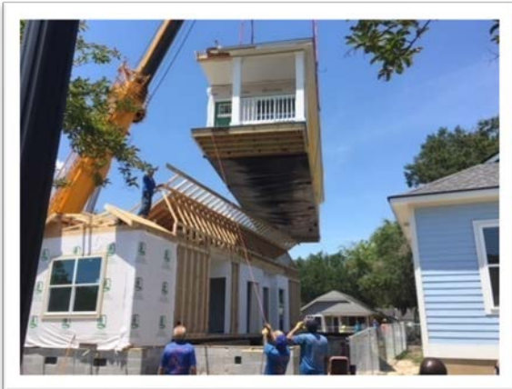
Above left, two modular homes ordered by CHSA Development, Inc. were set at Savannah Gardens on Pennsylvania Avenue on May 17, 2021-- marking the next step in CHSA's exploration of modular homes.
