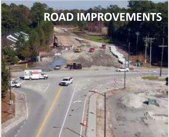
Road widenings, intersection improvements, signal upgrades
