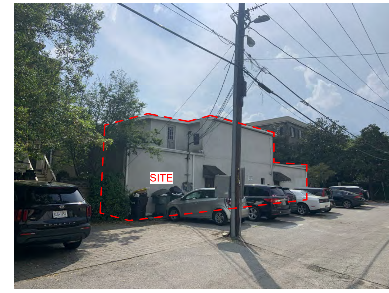
D. NORTHEAST CORNER E YORK LN. CONTEXT
