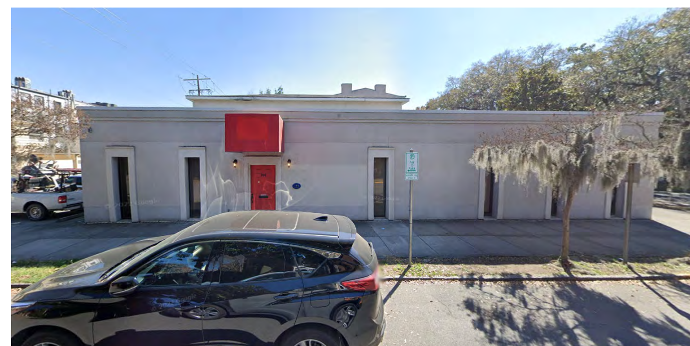
C. SITE VIEW FROM LINCOLN ST.
