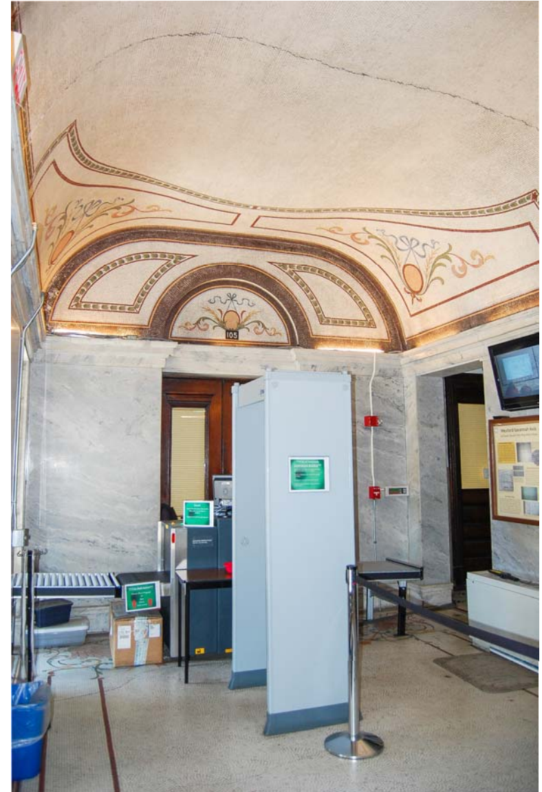
Interior of Lobby looking west, showing security equipment and television. Figure 27
