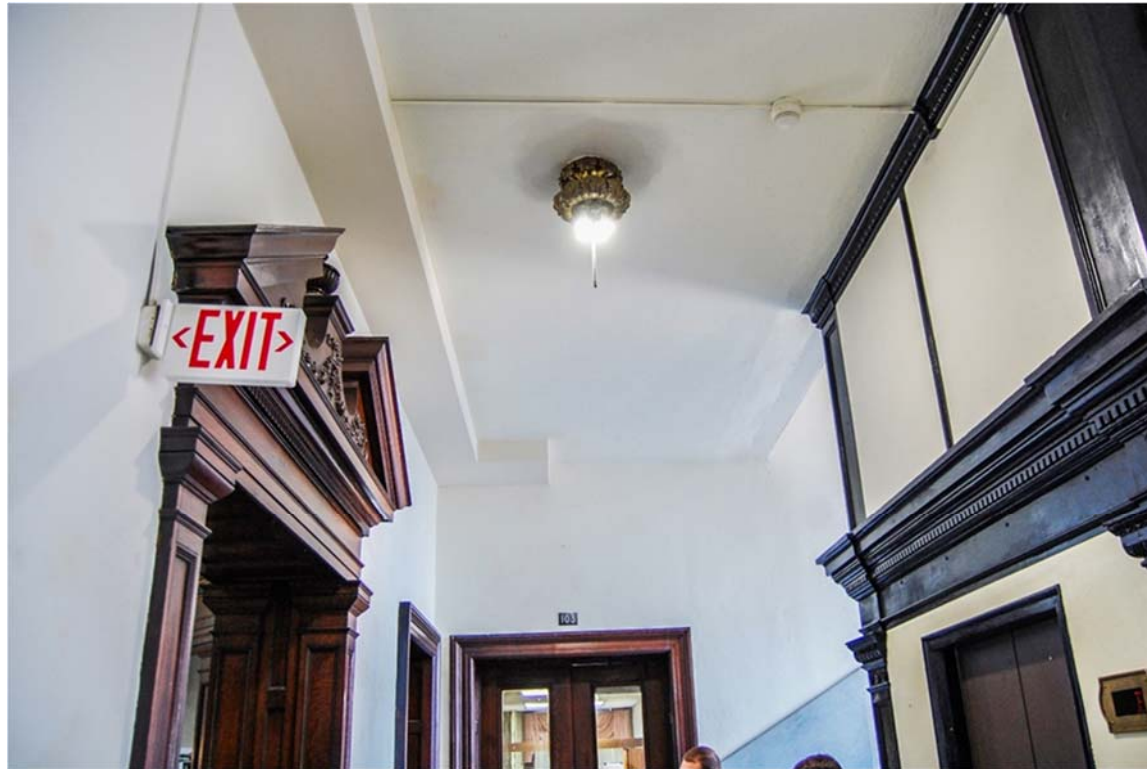
Ceiling of First Floor Corridor, looking west. Figure 12
