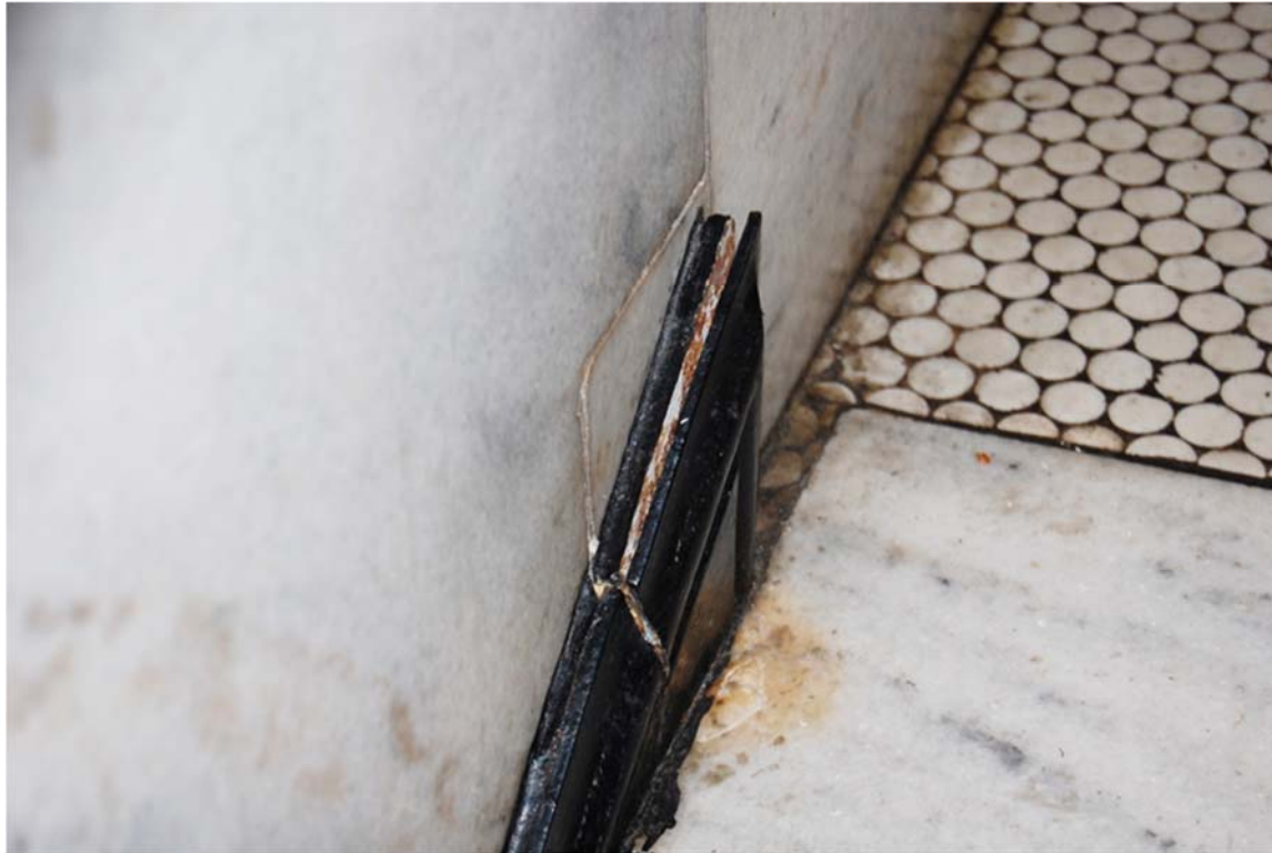
Detail of wood trim at side of Stair. Figure 14
