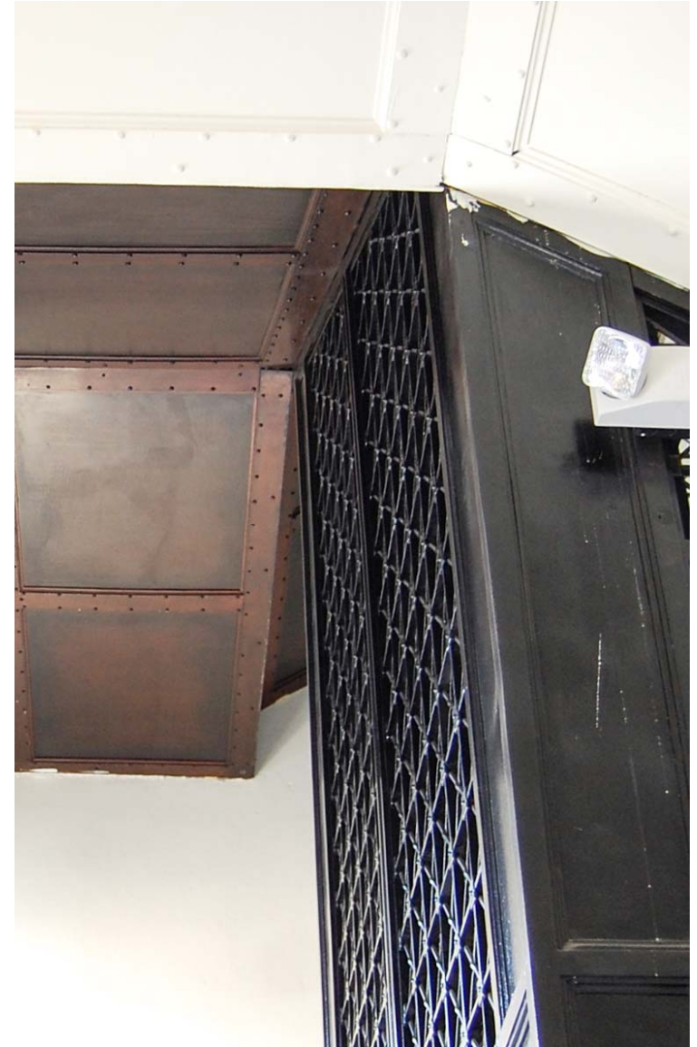
Contrasting faux finish and cream colored paint on Stair ceiling. Figure 59
