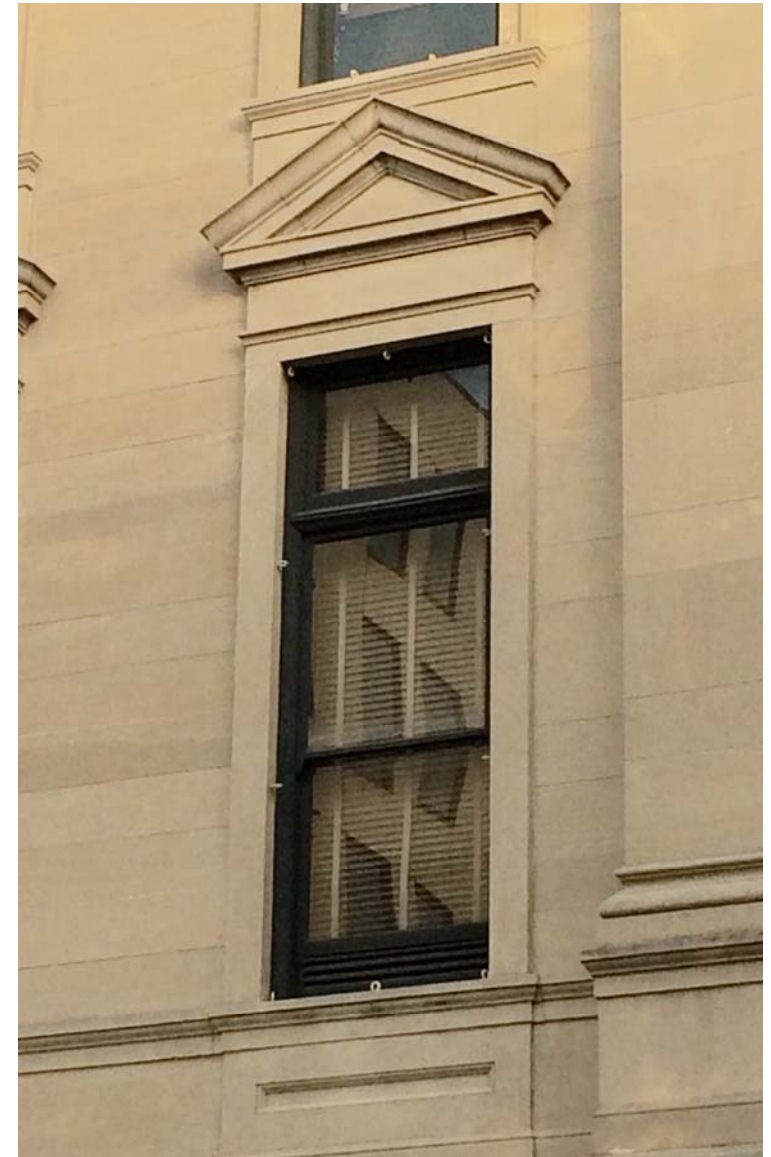
Exterior view of Council Chamber windows.
