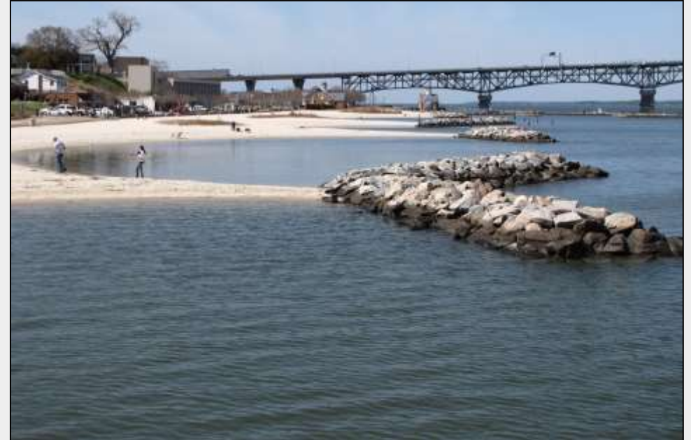
Example) A series of breakwaters promoting sediment accretion at Colonial National Historic Park, Virginia.
