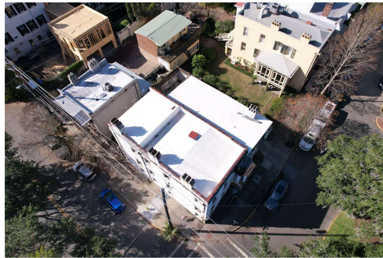
AERIAL VIEW FROM NE CORNER
