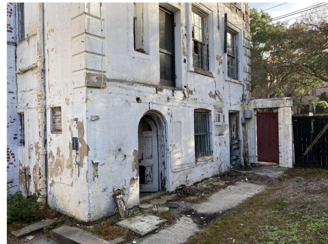
VIEW OF SOUTH FACADE & ABERCORN GATE FROM REAR YARD
