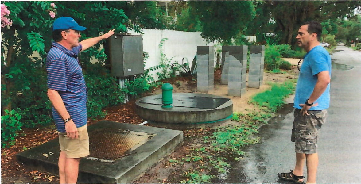
Figure 1. Project members Alan Robertson and Alfie Vick inspect drainage near critical infrastructure.
