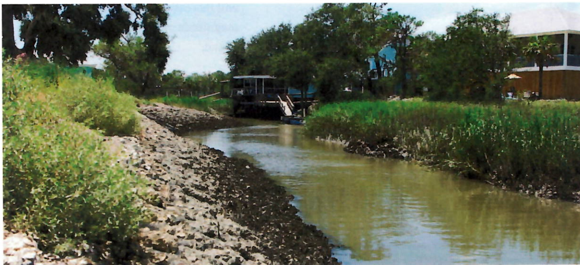
Figure 1.2. An example of natural infrastructure is the living shoreline located at the UGA Burton 4-H Center on Tybee Island.
