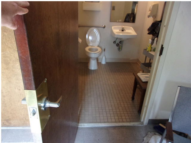
67. 555 West Bay Street Office - Women's staff restroom - Replace common restroom accessories (Non-Critical Repair)
