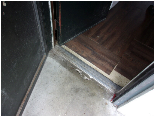
260-268 Yamacraw Village - Unit 261 - 1-bed/ 1-bath - HC unit - Low threshold at front door
