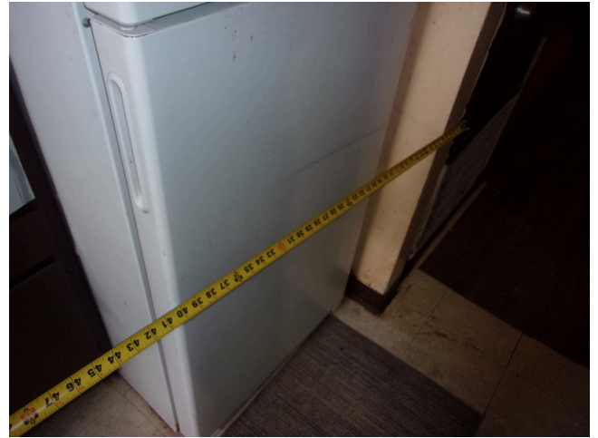
38. 260-268 Yamacraw Village - Unit 261 - 1-bed/ 1-bath - HC unit - Clear floor space at refrigerator
