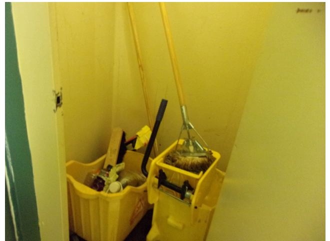
136. 349 West Bryan Street - Community center - Inspect fire extinguishers annually (Critical Repair)
