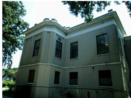
349 West Bryan Street - West elevation
