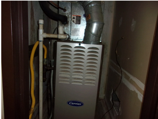
121-128 Yamacraw Village - Unit 126 - 2-bed/ 1-bath TH - Replace gas furnace (Non-Critical Repair)
