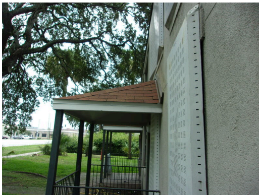
Porch roof view
