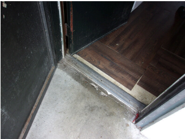
31. 260-268 Yamacraw Village - Unit 261 - 1-bed/ 1-bath - HC unit - Low threshold at front door
