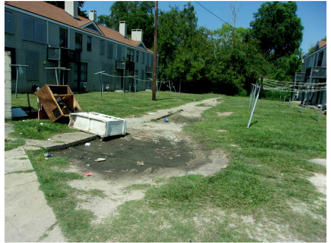
30. View of concrete walkway between apartment buildings
