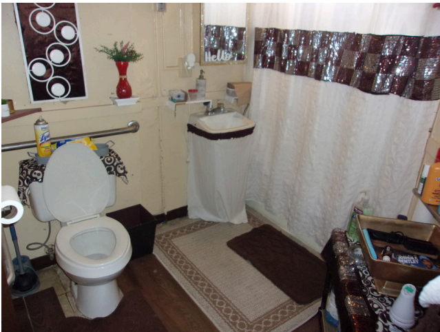
47. 260-268 Yamacraw Village - Unit 261 - 1-bed/ 1-bath - HC unit - Bathroom view, toilet with grab bars
