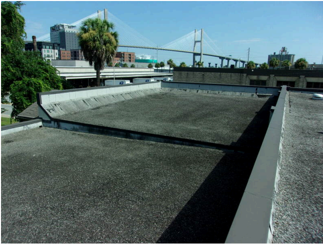
93. 555 West Bay Street built-up roofing view
