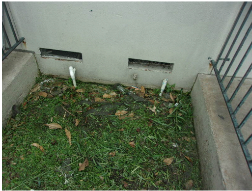
Crawl space vents
