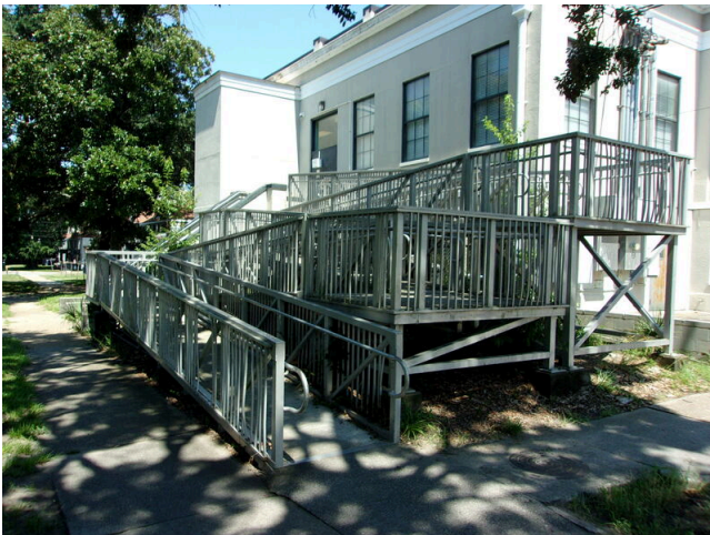
47. Metal ramp at rear of 349 West Bryan Street
