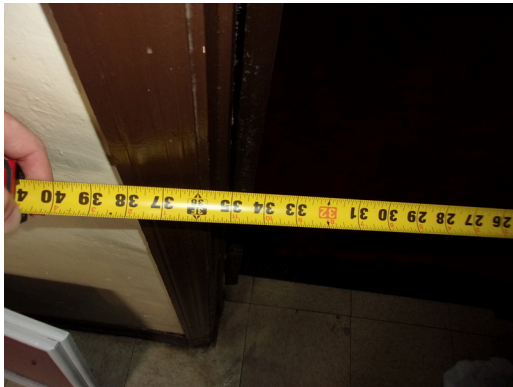
260-268 Yamacraw Village - Unit 261 - 1-bed/ 1-bath - HC unit - 34 inch clear opening at bedroom door
