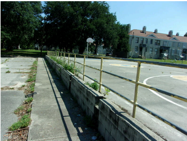
35. Refurbish and paint steel railing at basketball court (Non-Critical Repair)
