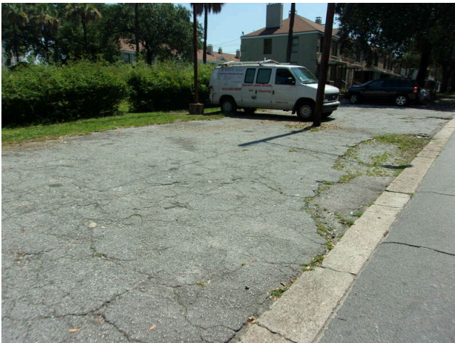
43. Replace and restripe asphalt parking surfaces (Non-Critical Repair)
