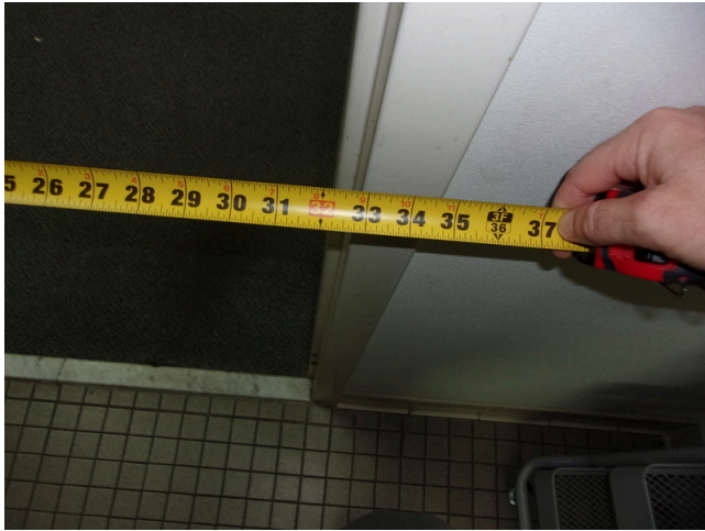
81. 555 West Bay Street Office - Men's public restroom - 32 inch clear opening at door
