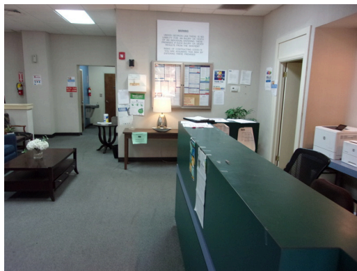
555 West Bay Street Office - Replace old carpet flooring (Non-Critical Repair)
