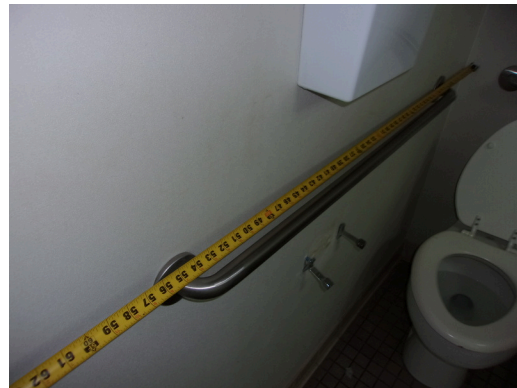
555 West Bay Street Office - Women's public restroom - Compliant side grab bar
