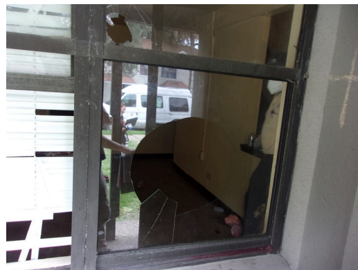
260-268 Yamacraw Village - Unit 264 - 2-bed/1-bath TH - Replace broken windows (Non-Critical Repair)
