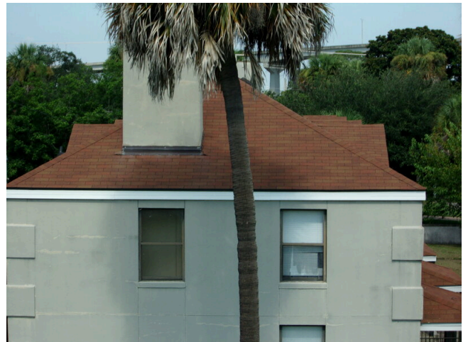
12. View of apartment building asphalt shingle roof
