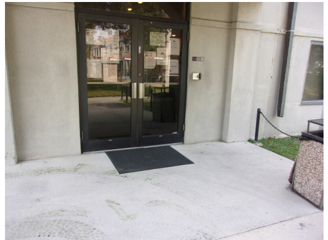
60. 555 West Bay Street Office - Main entry doors
