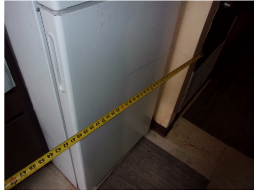
260-268 Yamacraw Village - Unit 261 - 1-bed/ 1-bath - HC unit - Clear floor space at refrigerator
