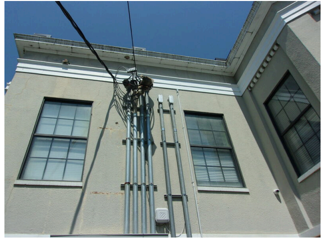
158. Electrical weather head and aluminum windows at 349 West Bryan Street
