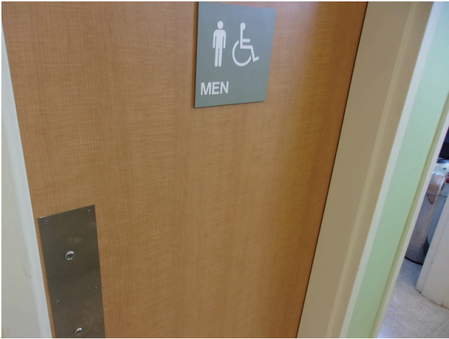
109. 349 West Bryan Street - 2nd floor Doctor's office - Men's public restroom - ADA signage
