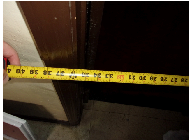
56. 260-268 Yamacraw Village - Unit 261 - 1-bed/ 1-bath - HC unit - 34 inch clear opening at bedroom door
