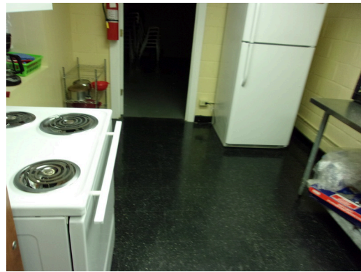
349 West Bryan Street - Community center - Replace old vinyl flooring (Non-Critical Repair)
