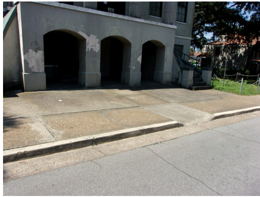
Repair and wash stucco siding at 349 West Bryan Street (Non-Critical Repair)
