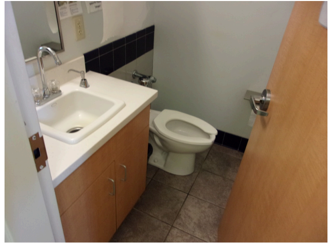
118. 349 West Bryan Street - 2nd floor Doctor's office - Staff restroom view
