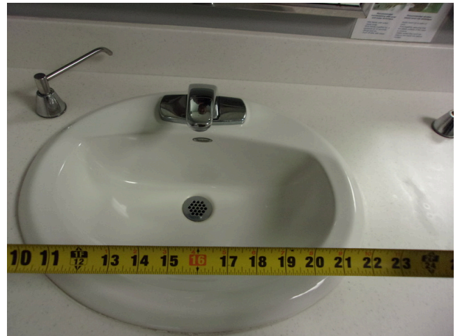
112. 349 West Bryan Street - 2nd floor Doctor's office - Men's public restroom - Clear floor space at sinks
