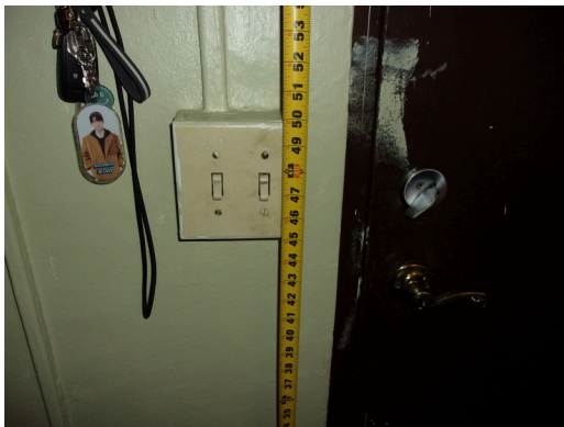
260-268 Yamacraw Village - Unit 261 - 1-bed/ 1-bath - HC unit - Light switch at 48 inches AFF
