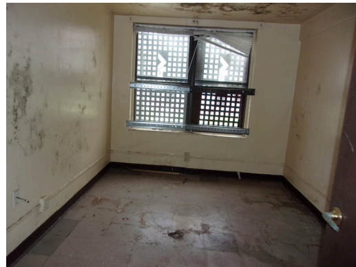
460-467 Yamacraw Village - Unit 461 - 1-bed/ 1-bath - HC unit/Down unit - Bedroom view
