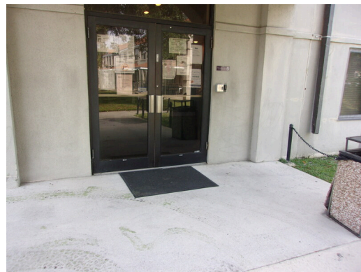
555 West Bay Street Office - Main entry doors
