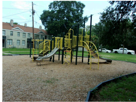
Playground equipment is past its EUL (Non-Critical Repair)
