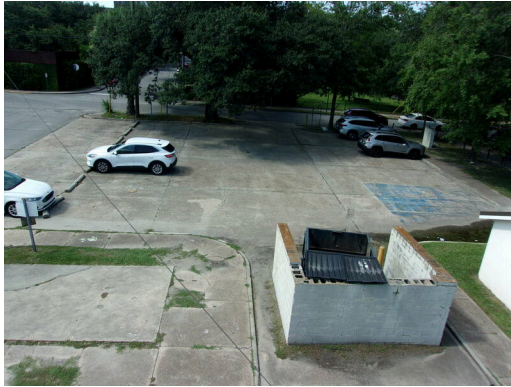
View of 555 West Bay Street concrete parking lot
