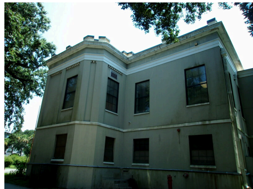
349 West Bryan Street - West elevation
