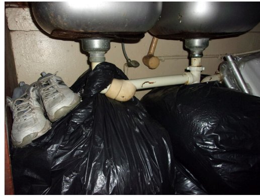
260-268 Yamacraw Village - Unit 261 - 1-bed/ 1-bath - HC unit - No scald and abrasion at sink
