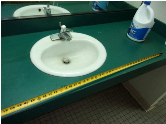
83. 555 West Bay Street Office - Men's public restroom - Clear floor space at levered sink
