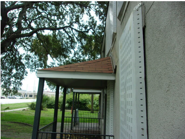
3. Porch roof view
