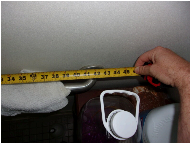
79. 555 West Bay Street Office - Women's public restroom - Compliant rear grab bar
