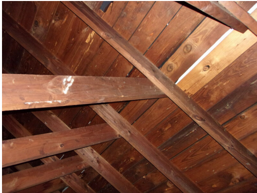
View of wood roof framing and decking
