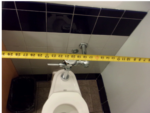
349 West Bryan Street - 2nd floor Doctor's office - Men's public restroom - ADA signage
