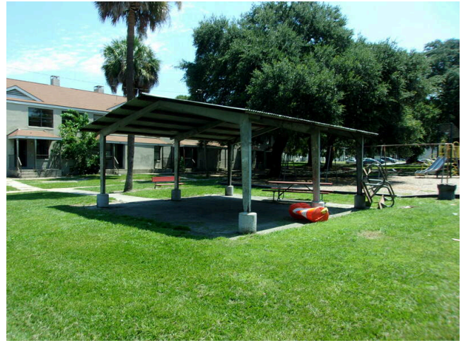
50. Metal gazebo view
