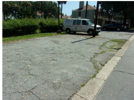
Replace and restripe asphalt parking surfaces (Non-Critical Repair)
