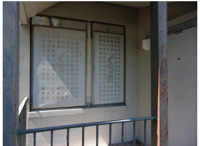
24. Typical metal window coverings for a down unit
