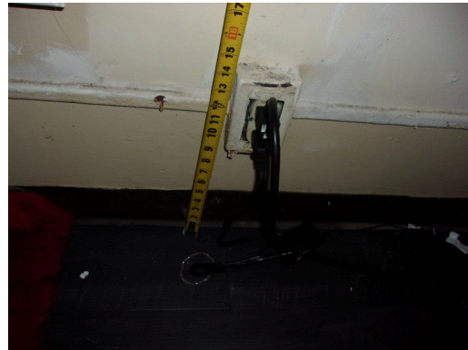
260-268 Yamacraw Village - Unit 261 - 1-bed/ 1-bath - HC unit - Outlet at 12 inches AFF
