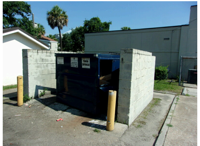
56. Replace CMU dumpster enclosures (Non-Critical Repair)
