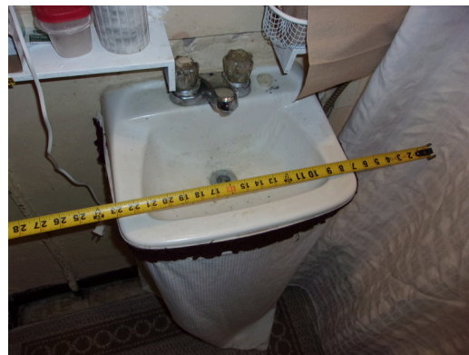
260-268 Yamacraw Village - Unit 261 - 1-bed/ 1-bath - HC unit - Clear floor space at roll-under sink
