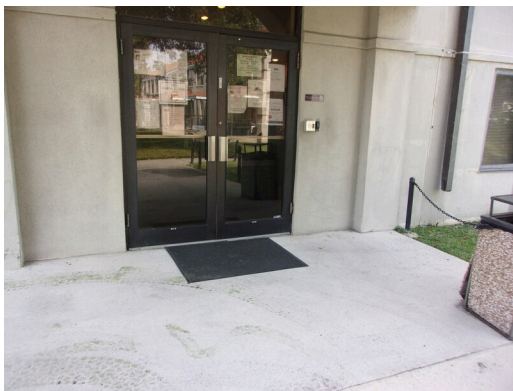
555 West Bay Street Office - Main entry doors
