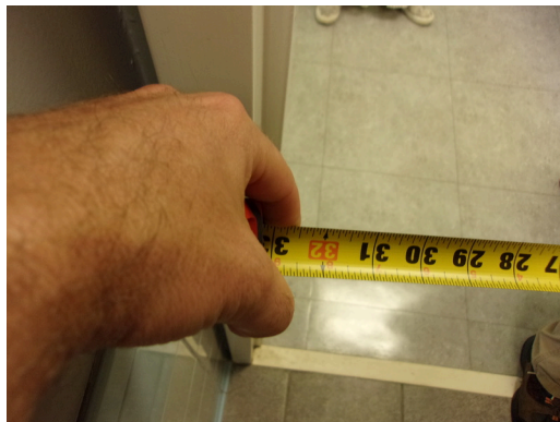
349 West Bryan Street - 2nd floor Doctor's office - Women's public restroom - 33 inch clear opening at door
