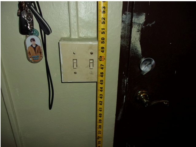
35. 260-268 Yamacraw Village - Unit 261 - 1-bed/ 1-bath - HC unit - Light switch at 48 inches AFF
