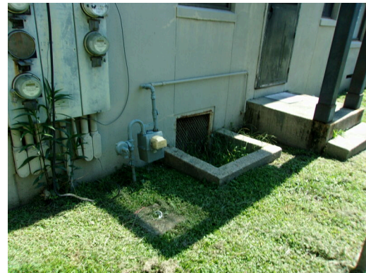
Crawlspace access door
