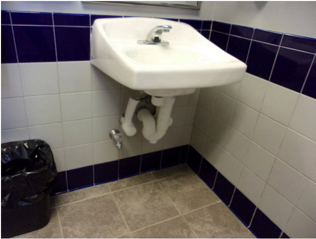
117. 349 West Bryan Street - 2nd floor Doctor's office - Men's public restroom - Scald and abrasion at sink
