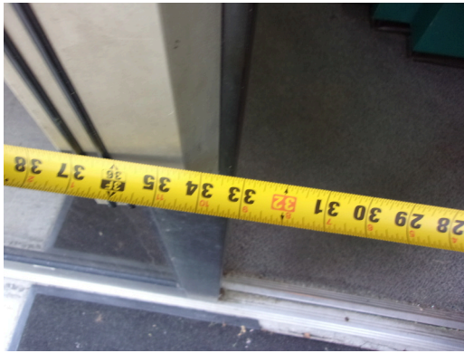
555 West Bay Street Office - 33 inch clear opening at main entry doors
