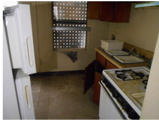
460-467 Yamacraw Village - Unit 460 - 1-bed/ 1-bath - Down unit - Kitchen view
