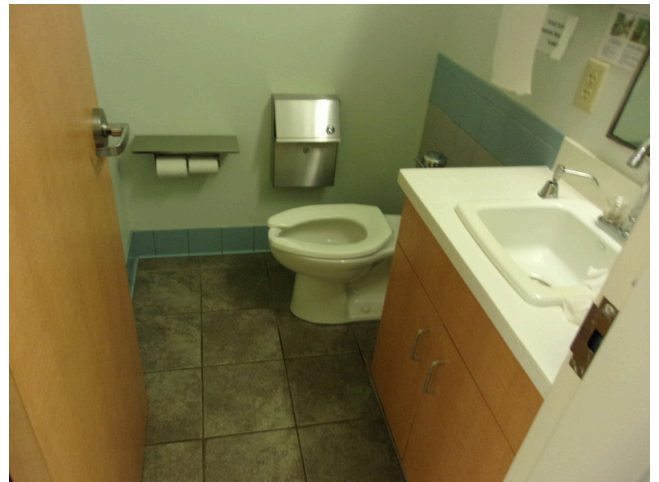
120. 349 West Bryan Street - 2nd floor Doctor's office - Staff restroom view
