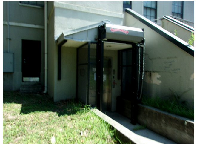
48. 349 West Bryan Street - Commercial overhead door
