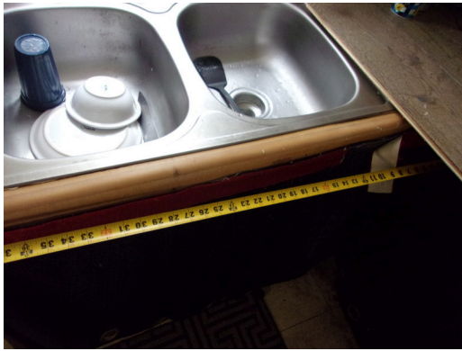
260-268 Yamacraw Village - Unit 261 - 1-bed/ 1-bath - HC unit - Roll-under sink
