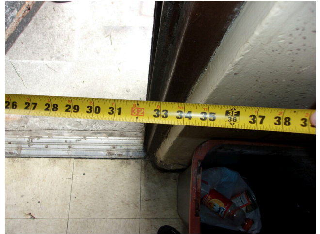
46. 260-268 Yamacraw Village - Unit 261 - 1-bed/ 1-bath - HC unit - 32 inch clear opening at rear door
