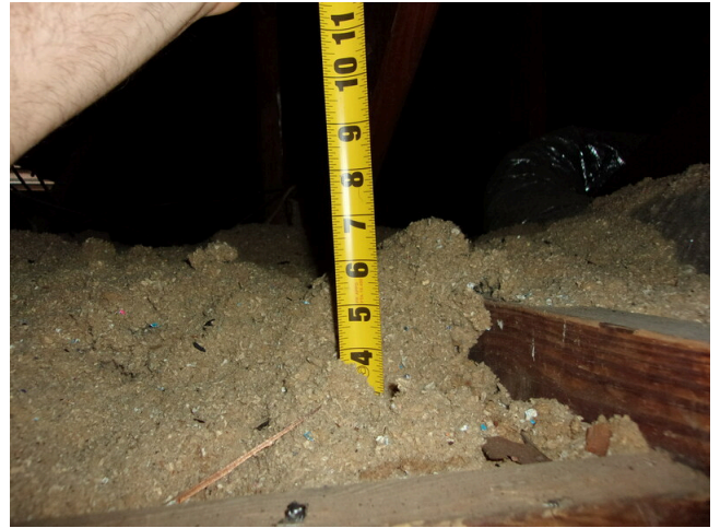
98. View of cellulose insulation in attic at 6 inches of depth
