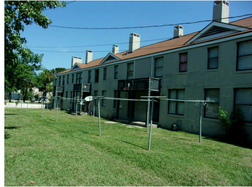
Apartment building rear elevation
