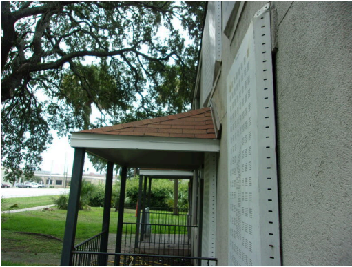
Porch roof view
