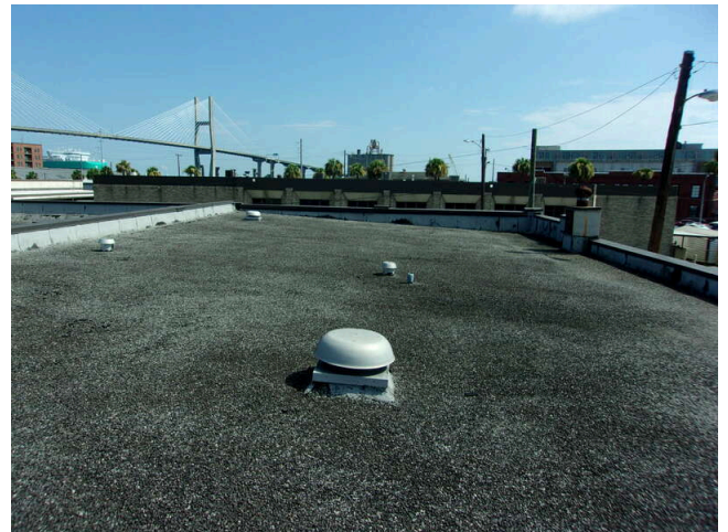
92. 555 West Bay Street built-up roofing view
