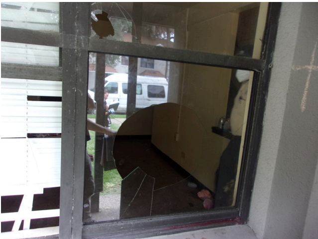
59. 260-268 Yamacraw Village - Unit 264 - 2-bed/ 1-bath TH - Replace broken windows (Non-Critical Repair)
