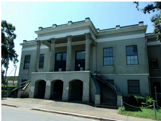
349 West Bryan Street - North elevation
