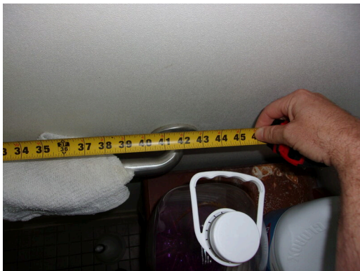
555 West Bay Street Office - Women's public restroom - Compliant rear grab bar
