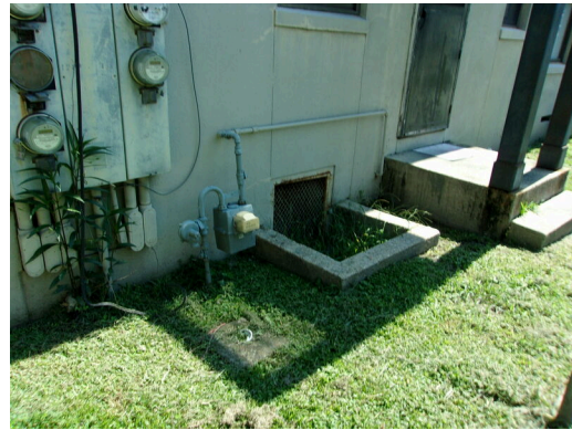
Crawlspace access door
