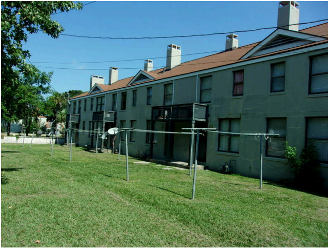
17. Apartment building rear elevation
