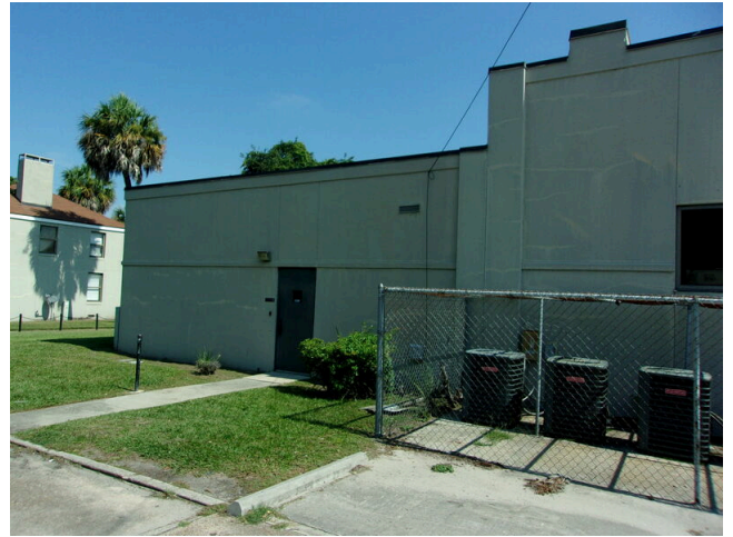
54. Chain link HVAC fencing
