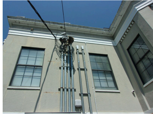
Electrical weather head and aluminum windows at 349 West Bryan Street
