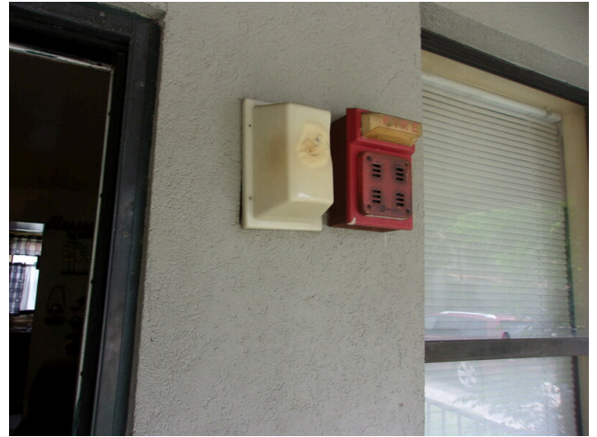
30. 260-268 Yamacraw Village - Unit 261 - 1-bed/ 1-bath - HC unit - Emergency call light and fire alarm
