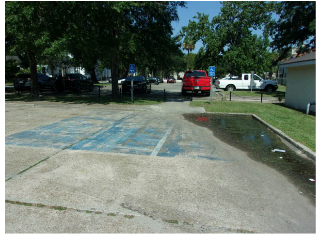
14. HC parking at 555 West Bay Street - Two (2) standard spaces, convert two (2) spaces to van accessible (Critical Repair)
