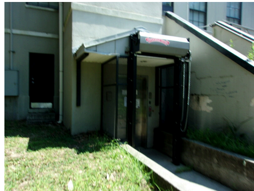
349 West Bryan Street - Commercial overhead door
