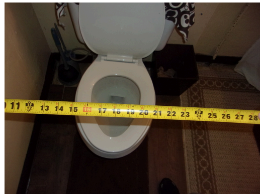
260-268 Yamacraw Village - Unit 261 - 1-bed/ 1-bath - HC unit - Clear floor space at toilet
