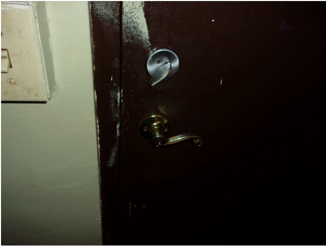
33. 260-268 Yamacraw Village - Unit 261 - 1-bed/ 1-bath - HC unit - Levered door hardware
