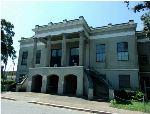
349 West Bryan Street - North elevation
