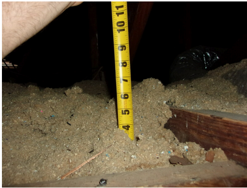
View of cellulose insulation in attic at 6 inches of depth
