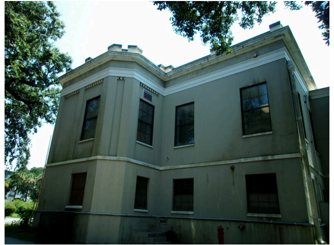
42. 349 West Bryan Street - West elevation
