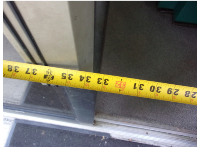
62. 555 West Bay Street Office - 33 inch clear opening at main entry doors
