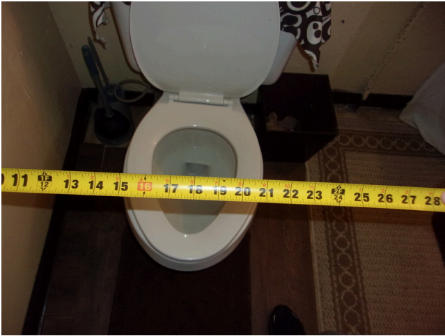
49. 260-268 Yamacraw Village - Unit 261 - 1-bed/ 1-bath - HC unit - Clear floor space at toilet
