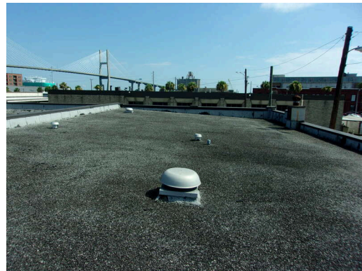
555 West Bay Street built-up roofing view
