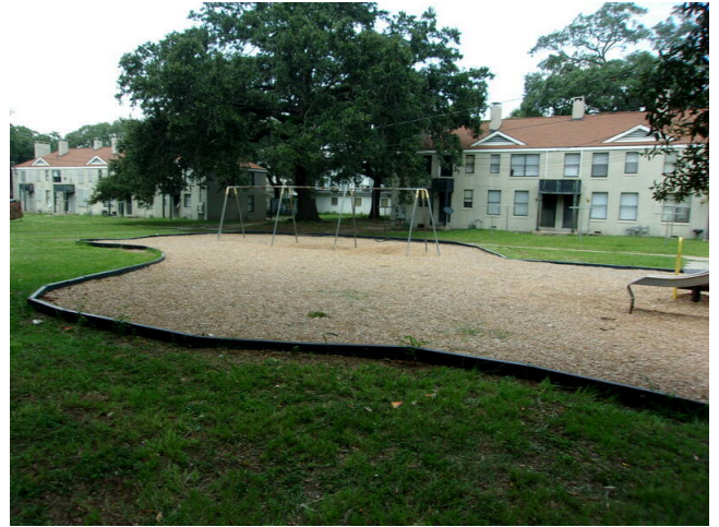
6. Playground equipment is past its EUL (Non-Critical Repair)
