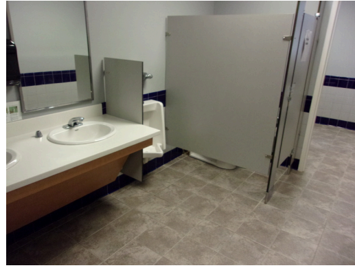
349 West Bryan Street - 2nd floor Doctor's office - Men's public restroom - Room view
