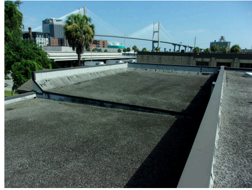
555 West Bay Street built-up roofing view
