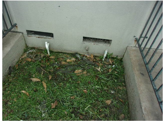
2. Crawl space vents
