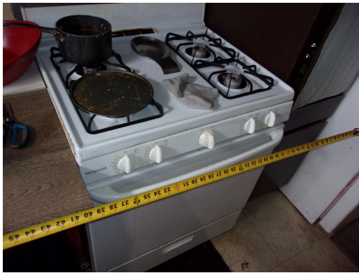
260-268 Yamacraw Village - Unit 261 - 1-bed/ 1-bath - HC unit - Clear floor space at range/ oven
