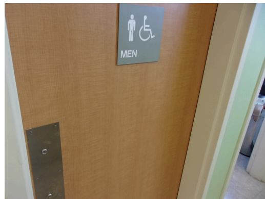
349 West Bryan Street - 2nd floor Doctor's office - Men's public restroom - ADA signage
