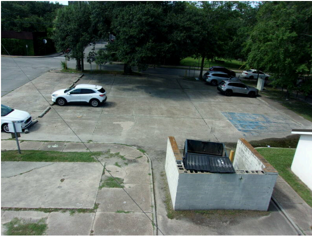
13. View of 555 West Bay Street concrete parking lot
