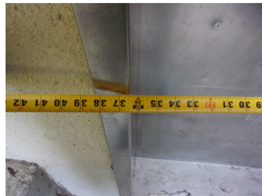
36 inch clear opening at elevator door
