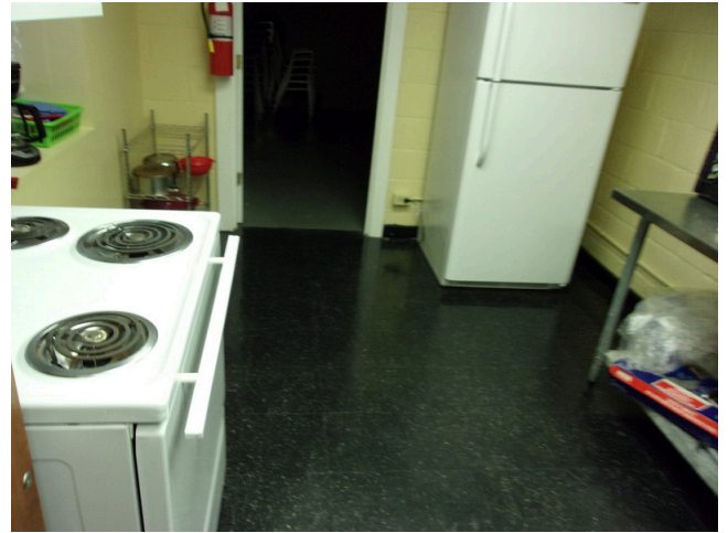
138. 349 West Bryan Street - Community center - Replace old vinyl flooring (Non-Critical Repair)
