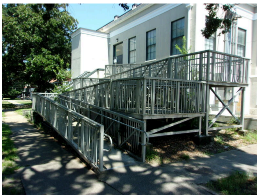
Metal ramp at rear of 349 West Bryan Street
