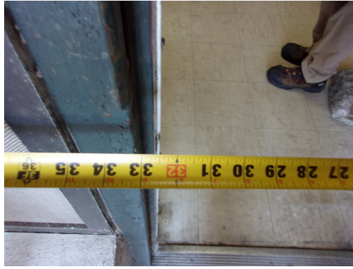
349 West Bryan Street - Community center - 32 inch clear opening at entry door
