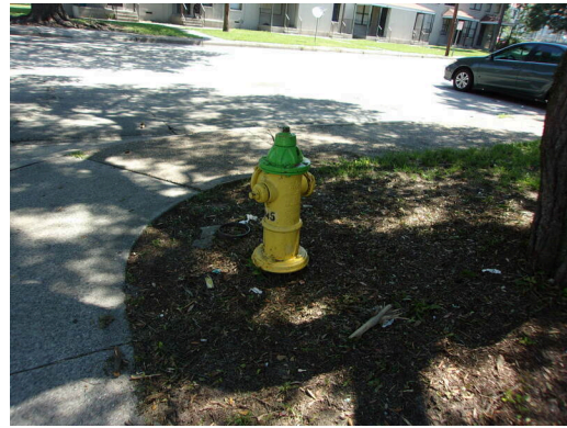
Fire hydrant near municipal street
