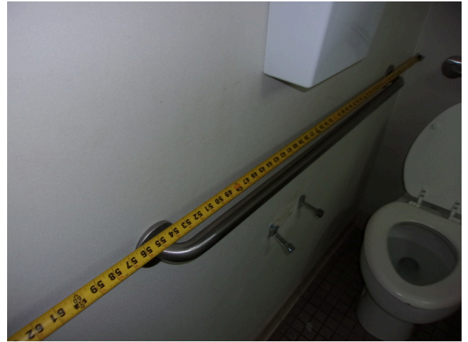
78. 555 West Bay Street Office - Women's public restroom - Compliant side grab bar
