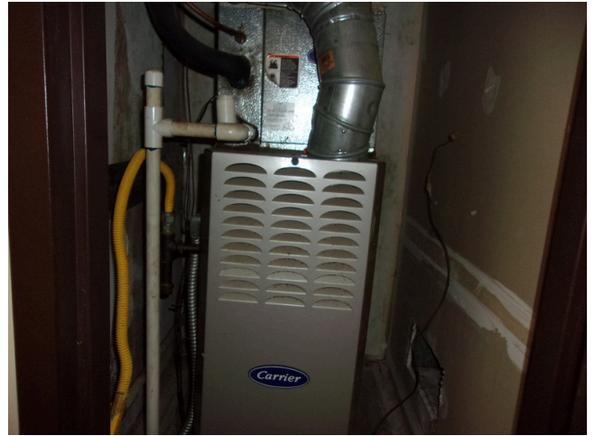
10. 121-128 Yamacraw Village - Unit 126 - 2-bed/ 1-bath TH - Replace gas furnace (Non-Critical Repair)
