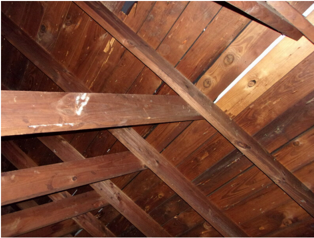
97. View of wood roof framing and decking
