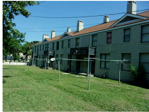
Apartment building rear elevation
