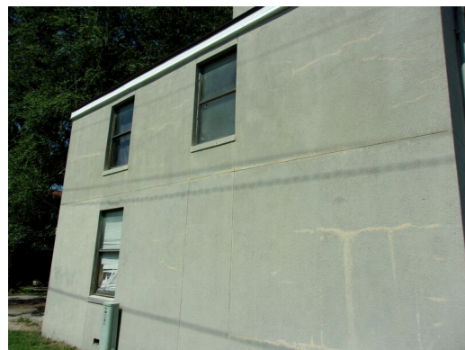
View of stucco siding
