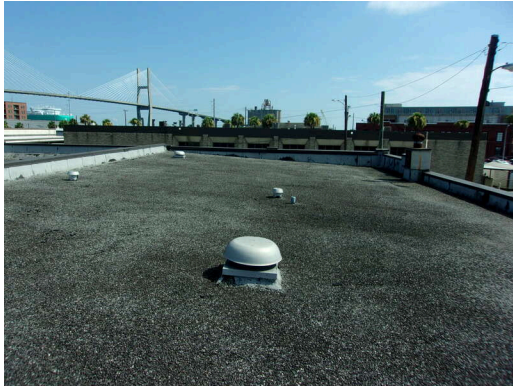
555 West Bay Street built-up roofing view
