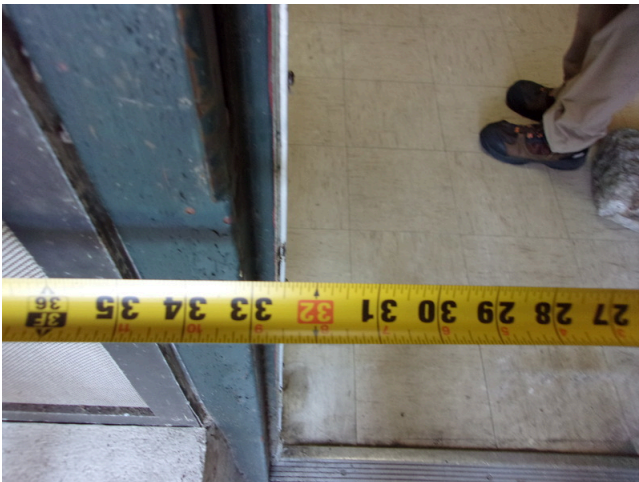
131. 349 West Bryan Street - Community center - 32 inch clear opening at entry door
