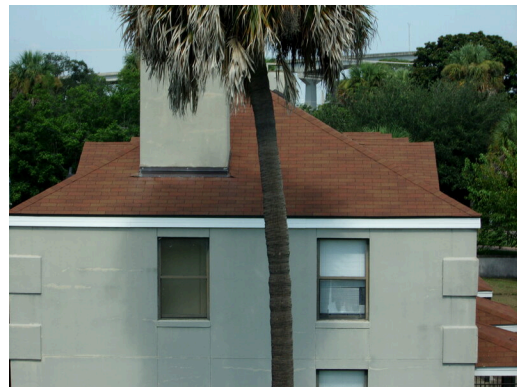
View of apartment building asphalt shingle roof
