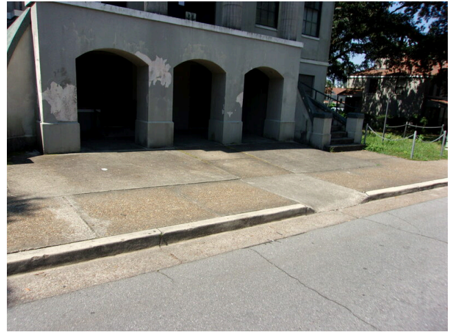
46. Repair and wash stucco siding at 349 West Bryan Street (Non-Critical Repair)
