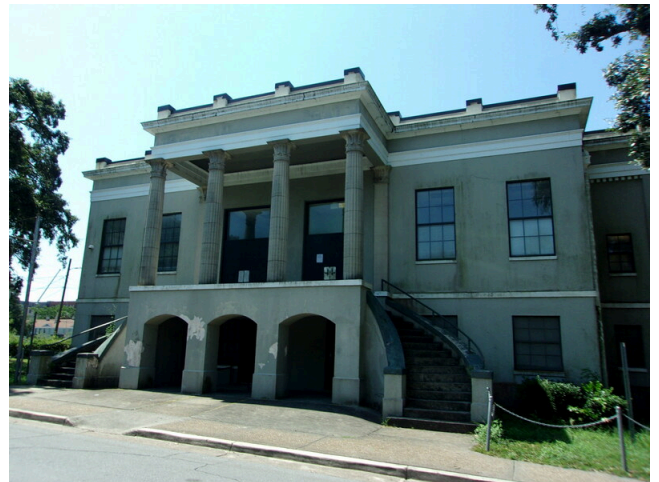
44. 349 West Bryan Street - North elevation
