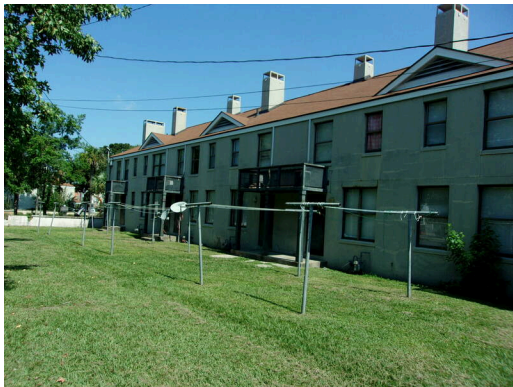
Apartment building rear elevation
