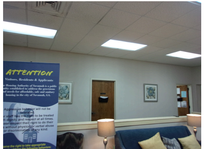
64. 555 West Bay Street Office - Acoustical ceiling tile view
