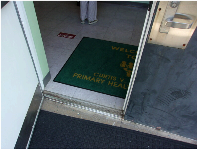
101. 349 West Bryan Street - 2nd floor Doctor's office - Low threshold at main entry door
