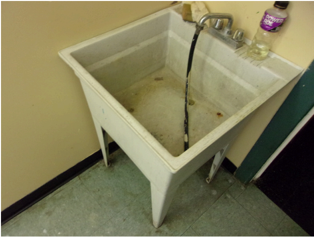
133. 349 West Bryan Street - Community center - Staff restroom - Replace common restroom accessories (Non-Critical Repair)
