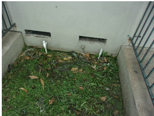
Crawl space vents
