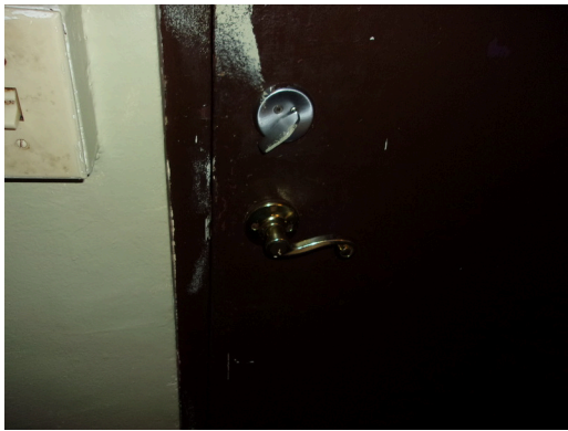
260-268 Yamacraw Village - Unit 261 - 1-bed/ 1-bath - HC unit - Levered door hardware
