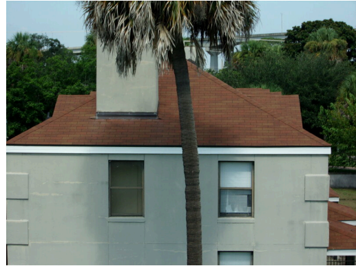
View of apartment building asphalt shingle roof
