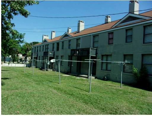
Apartment building rear elevation
