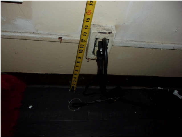
57. 260-268 Yamacraw Village - Unit 261 - 1-bed/ 1-bath - HC unit - Outlet at 12 inches AFF
