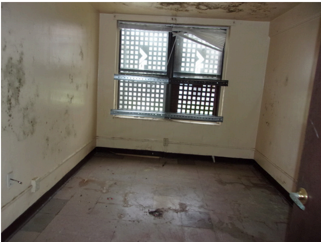
71. 460-467 Yamacraw Village - Unit 461 - 1-bed/ 1-bath - HC unit/Down unit - Bedroom view
