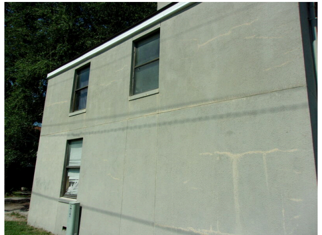
28. View of stucco siding
