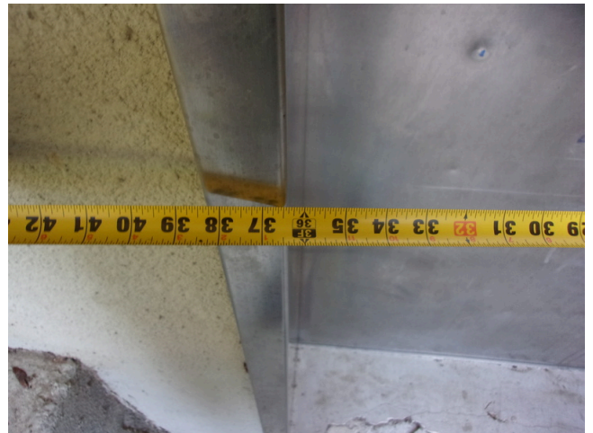
100. 36 inch clear opening at elevator door
