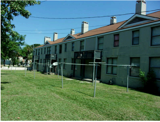
Apartment building rear elevation
