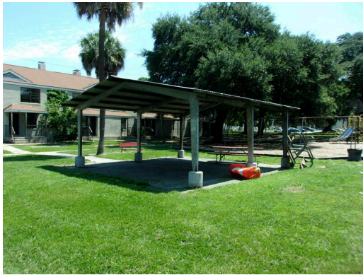
Metal gazebo view
