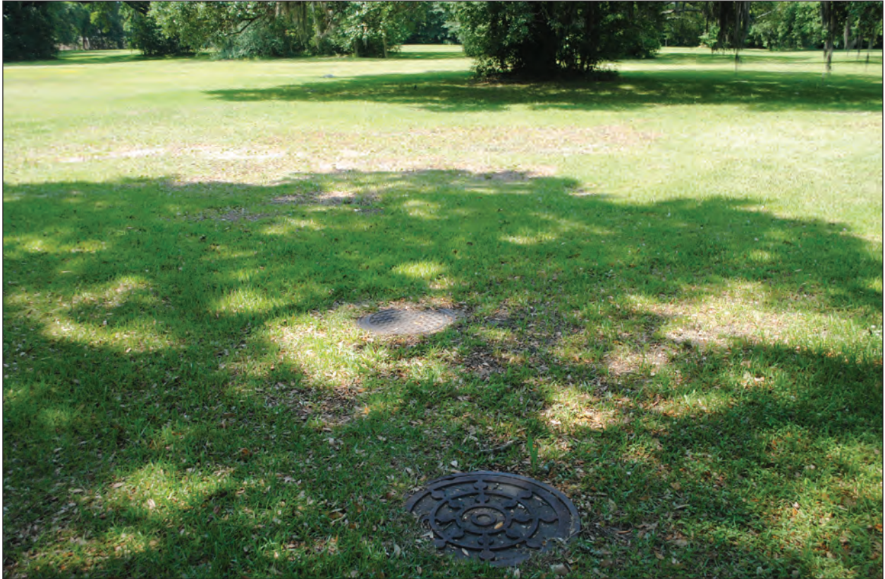
Figure 4.8 View of project tract and sewer line access within the project tract, facing south.
