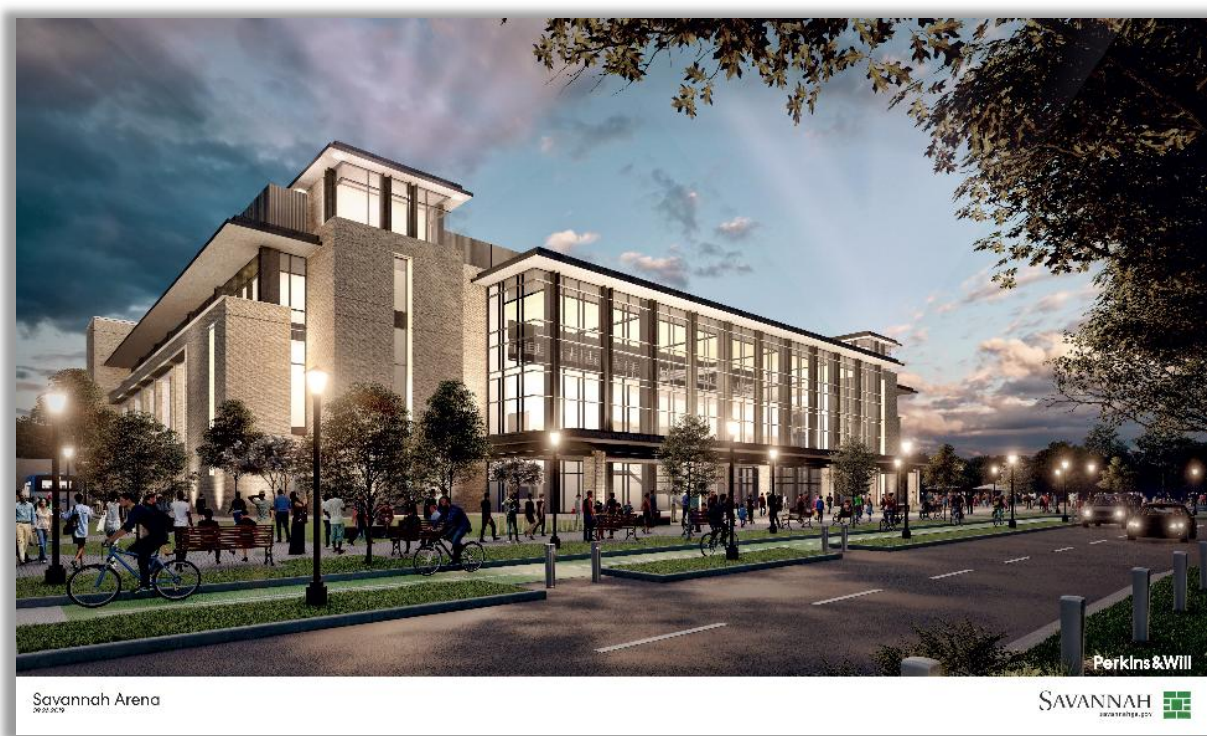
Rendering of Southwesterly View of Arena Under Construction
