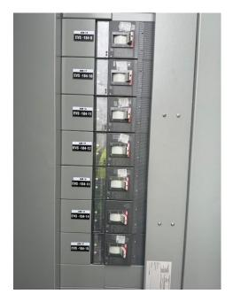
Note\*\*The breaker throw is heavy and should be immediately followed with a loud and obvious "clack"noise. The lock out cover should be able to cover the breaker and not allow movement. If the lock out cover does not sit flush the breaker is not in the off position. \*\*
