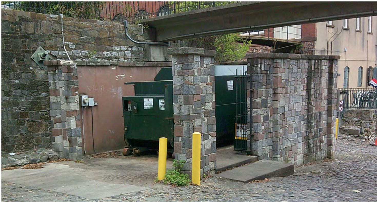
Trash enclosures without doors only partially conceal compactors from view, and their open top allows views down into the dirty enclosures from the bridges and walkways above.
