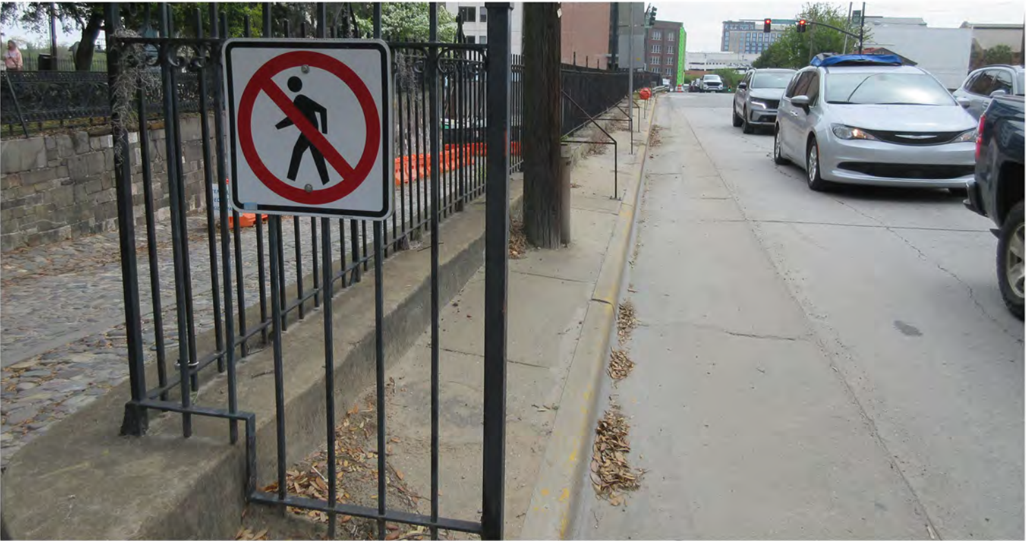
No safe pedestrian route along East Bay Street approaching East Broad Street.
