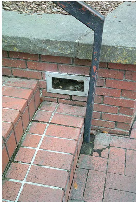
Broken footpath lights and bollard lights along the river.
