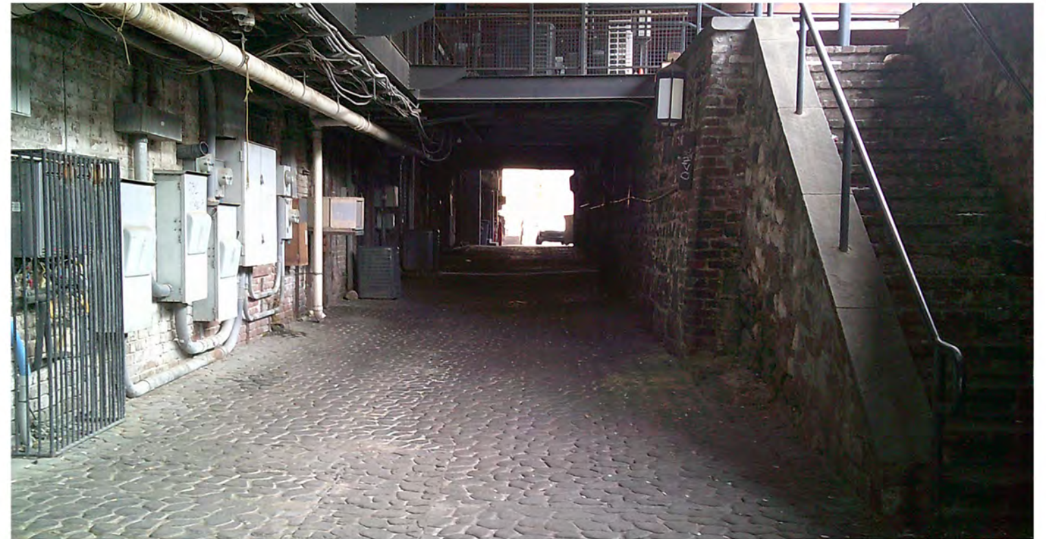
Poorly lit passages on Factors Walk appear uninviting and present a security risk.
