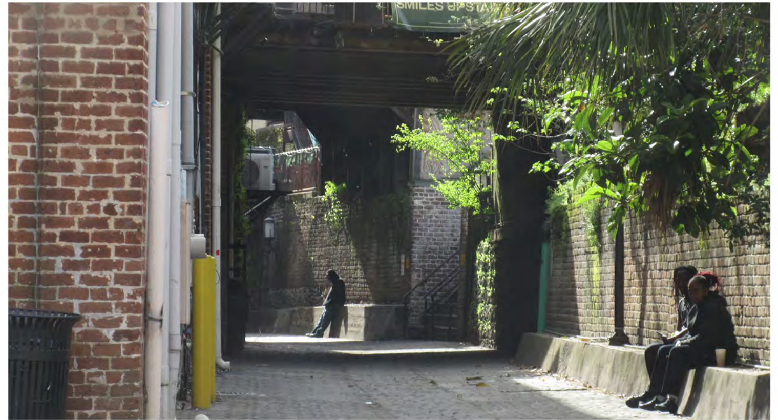
View east along Factors Walk showing vegetation growing from the masonry walls. These areas also lack smoking receptacles.
