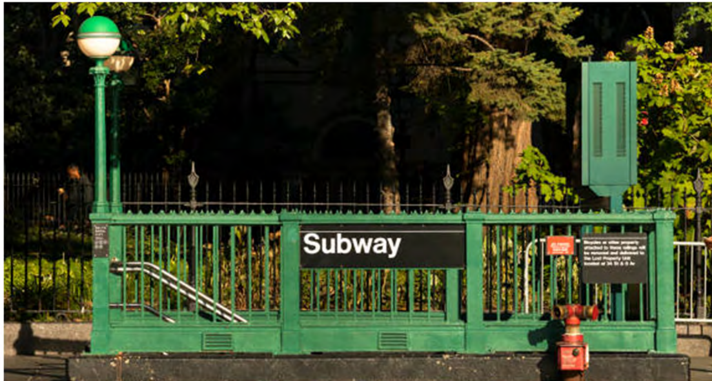
Stairways highlighted with distinctive lighting and color schemes provide orientation. (New York City, USA)
