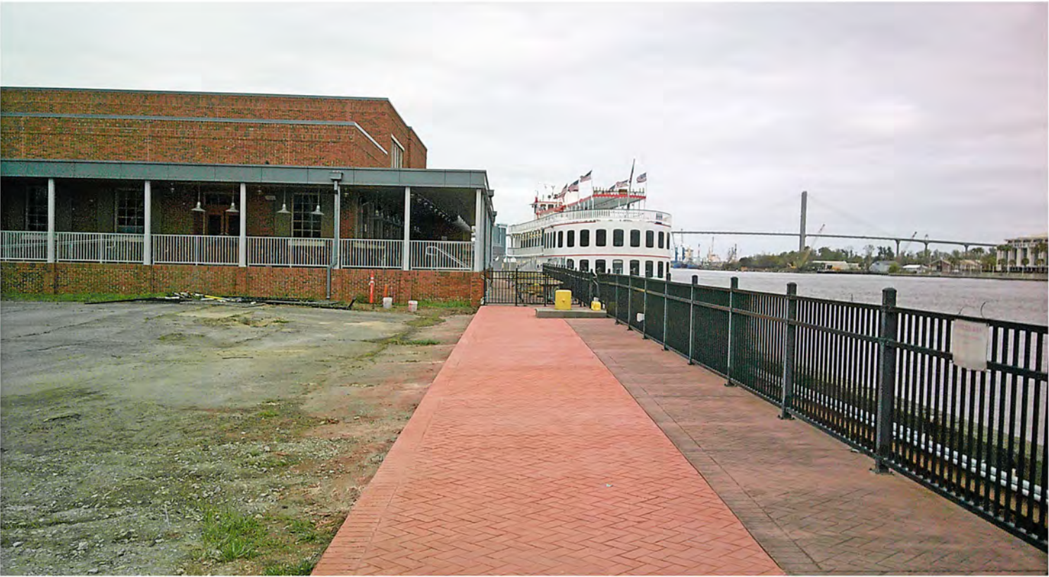
Discontinuity in the materials of the riverwalk and a distinct break in the line of movement along the river.
