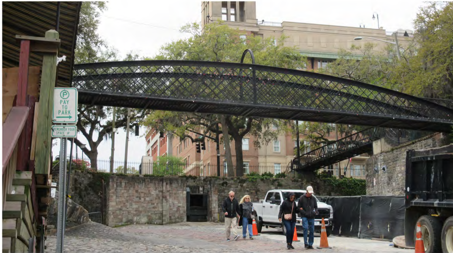
Bridges may present an opportunity to identify the name of ramp / street and to help with wayfinding.
