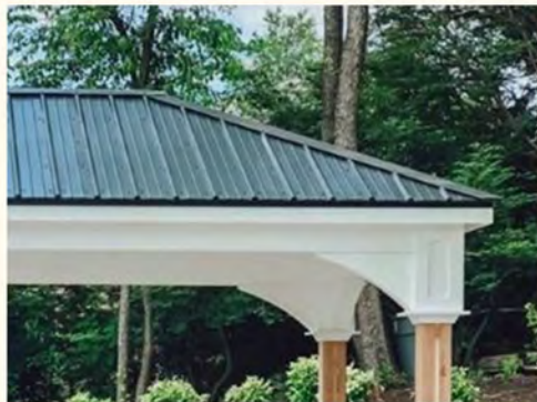
Raised, low slope roof over enclosure
