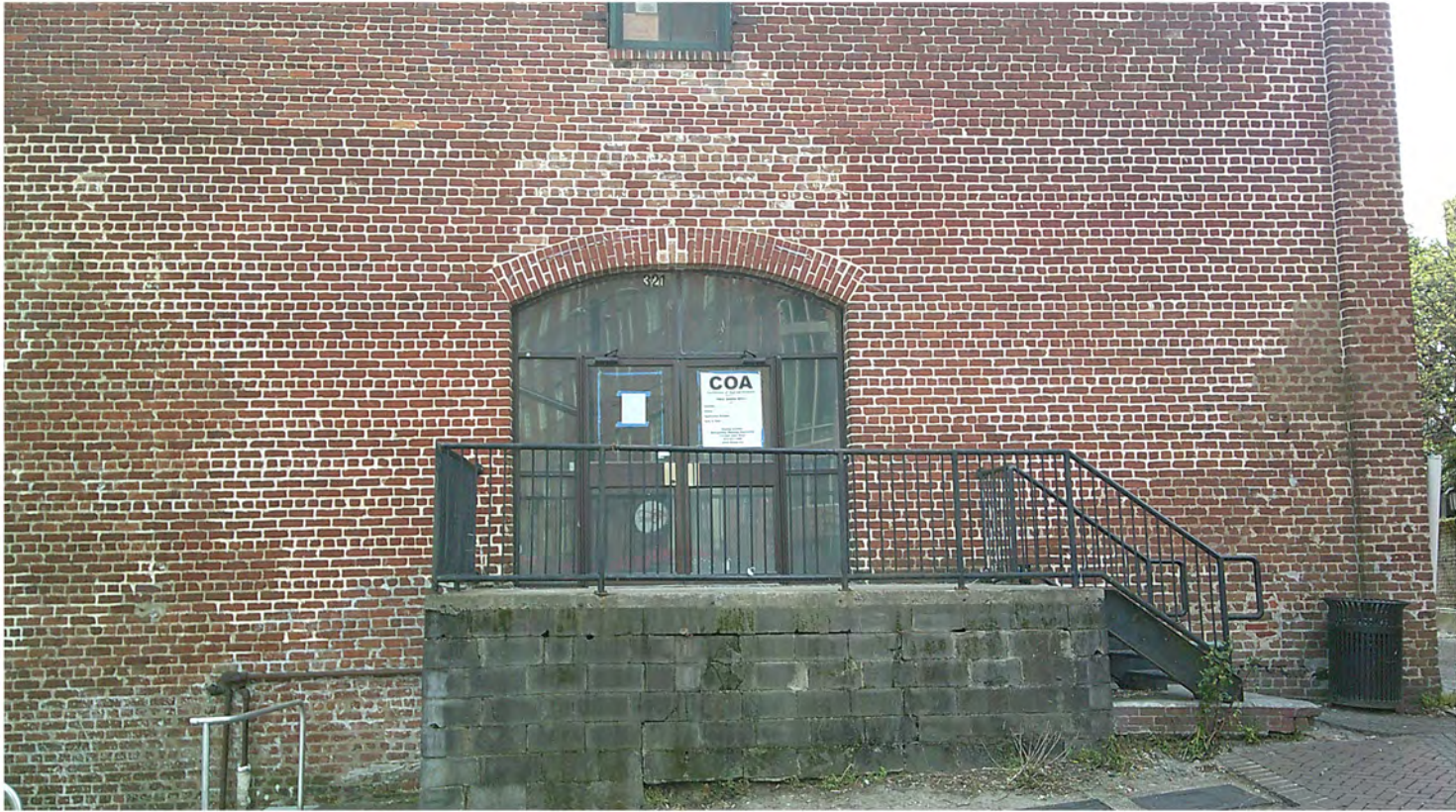
Buildings still in need of renovation are often the first impression for visitors coming down to River Street.
