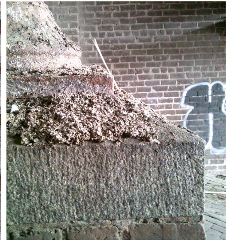
Many surfaces are in need of regular cleaning. These steps on the west end of River Street and columns under the Cotton Exchange have accumulated stains and grime due to a lack of consistent cleaning.
