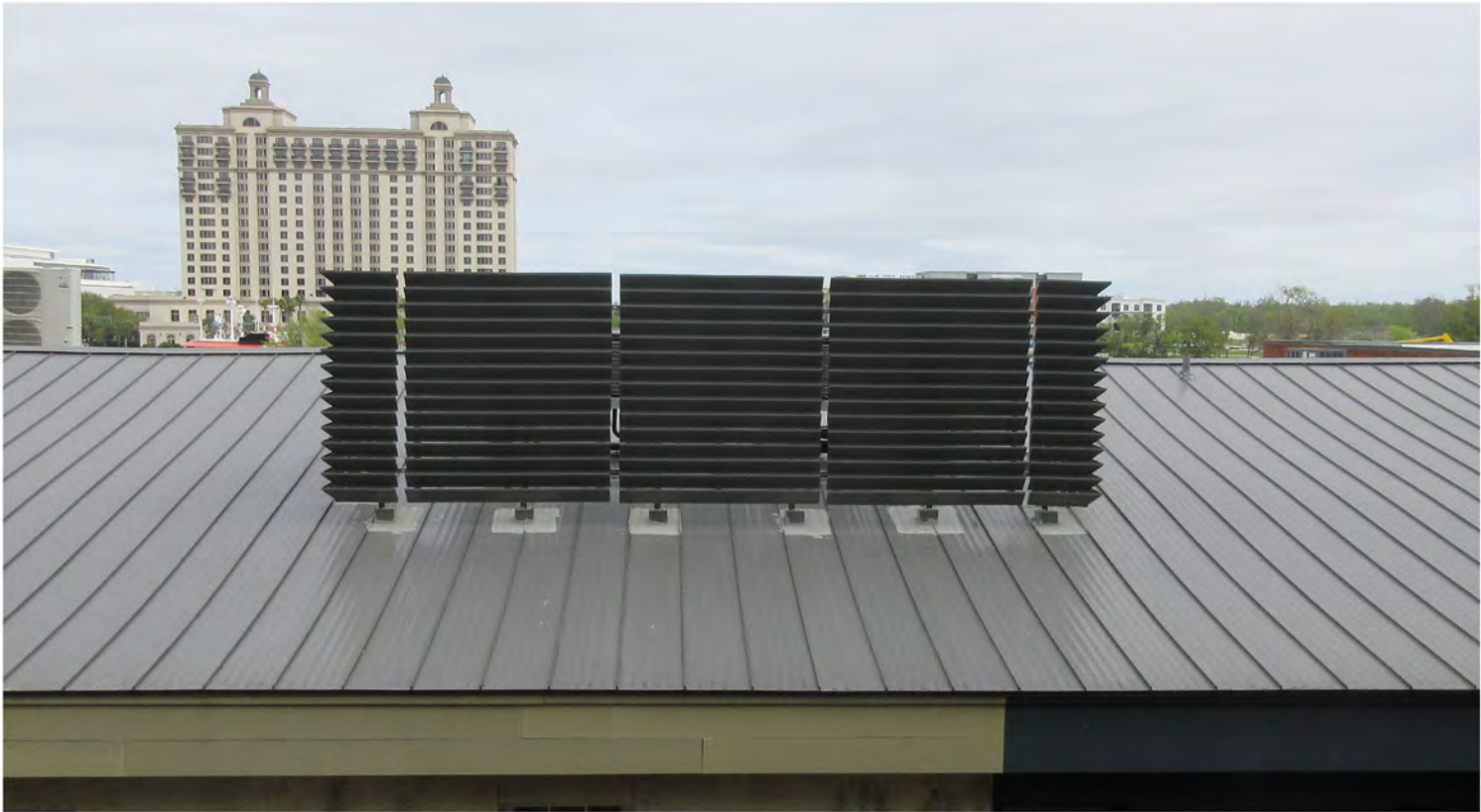
Utility screening, when applied, was observed to be an effective method of concealing unsightly rooftop units.
