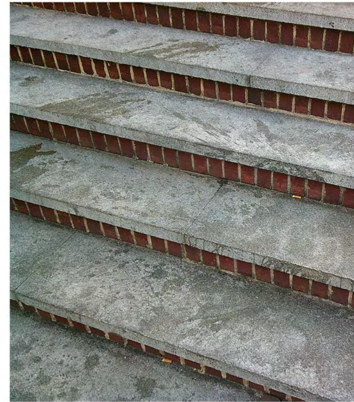
Many surfaces are in need of regular cleaning. These steps on the west end of River Street and columns under the Cotton Exchange have accumulated stains and grime due to a lack of consistent cleaning.
